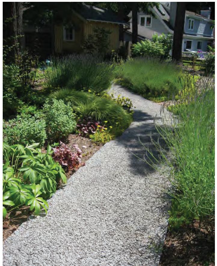
Pervious paving at a development in Kirkland.
