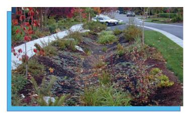
**Rain Gardens** slow the flow of rainwater runoff and let it filter into the ground naturally.
