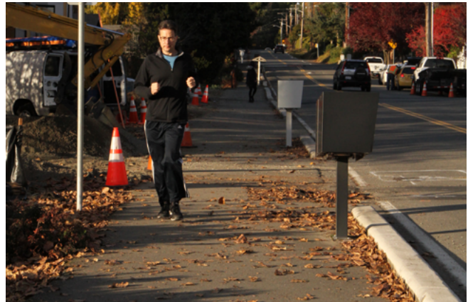
Figure 1.24: Extruded curb utilized by pedestrians (City of Kirkland).
