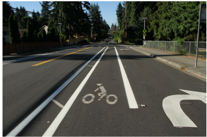
Figure 1.29: Buffered bike lane on 84th Ave NE (City of Kirkland).
