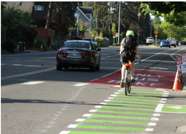
Figure 1.60: Green conflict zone markings extend the bike lane on Market St through the Juanita Bay Park intersection (City of Kirkland).
