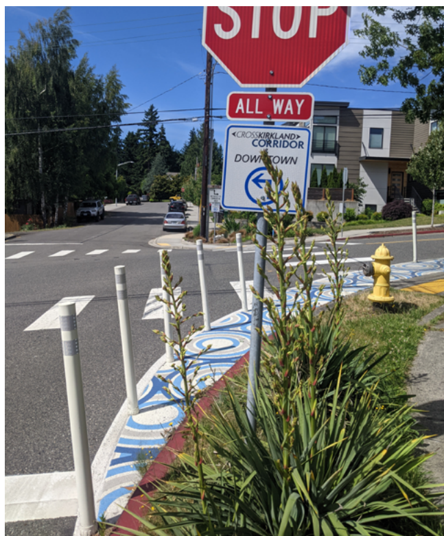
Figure 1.9: Curb bulbout with delineators and a CKC wayfinding sign at intersection of 114th Ave NE and NE 87th St (City of Kirkland).
