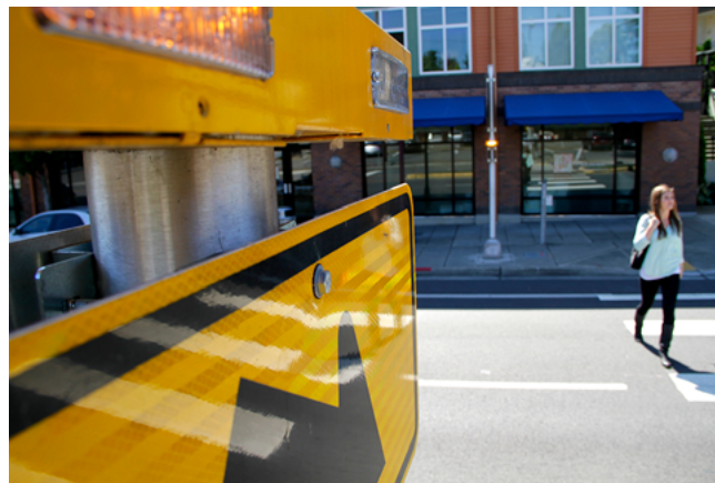
Figure 1.11: Rectangular Rapid Flashing Beacon (City of Kirkland).
