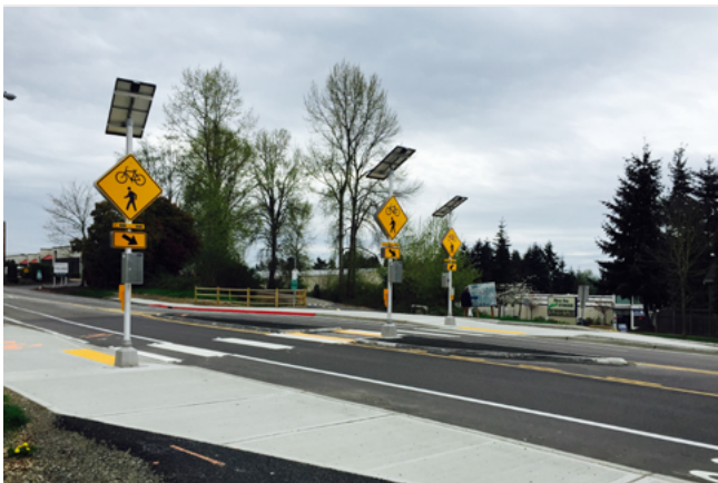
Figure 1.26: RRFBs on 6th St in Kirkland (City of Kirkland).
