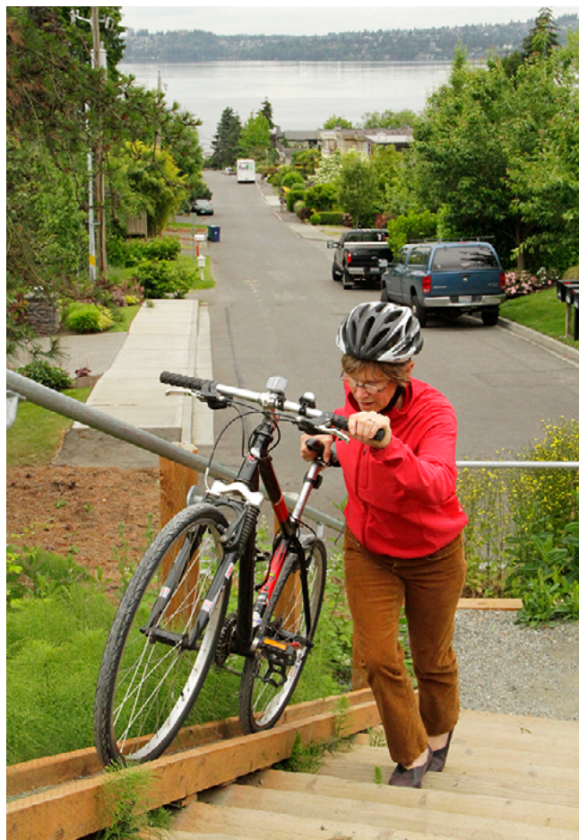
Figure 1.13: A runnel being used by a bicyclist onto the CKC (City of Kirkland).
