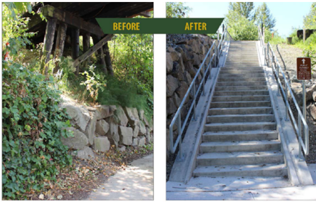
Figure 1.6: A stairway with bicycle runnel provides access to the CKC. This was completed as part of the Neighborhood Safety Program.
