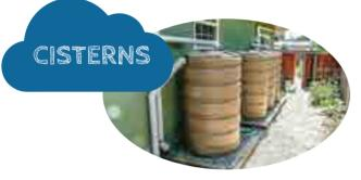
A cistern is a large, above-ground container used to collect roof water. During the winter, cisterns collect rain and slowly release it into the ground or your garden. In the summer, water can be collected and used for watering.
