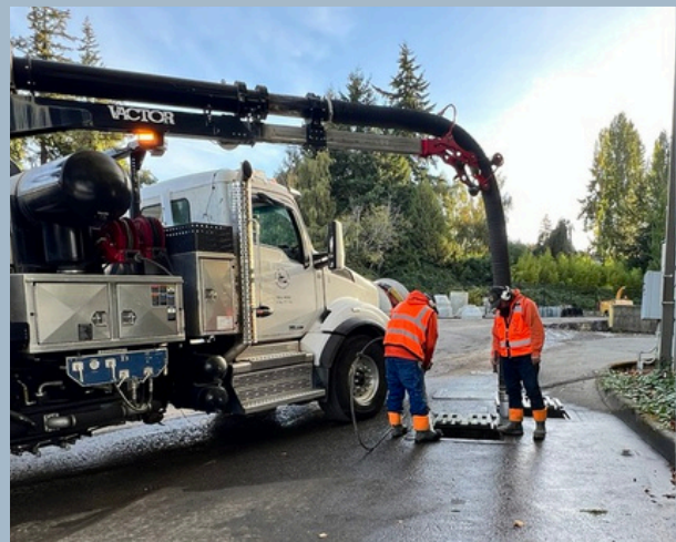
Above: Crews performing maintenance on a structure with City vactor truck.
