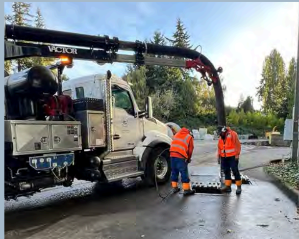
Above: Crews performing maintenance on a structure with City victor truck.
