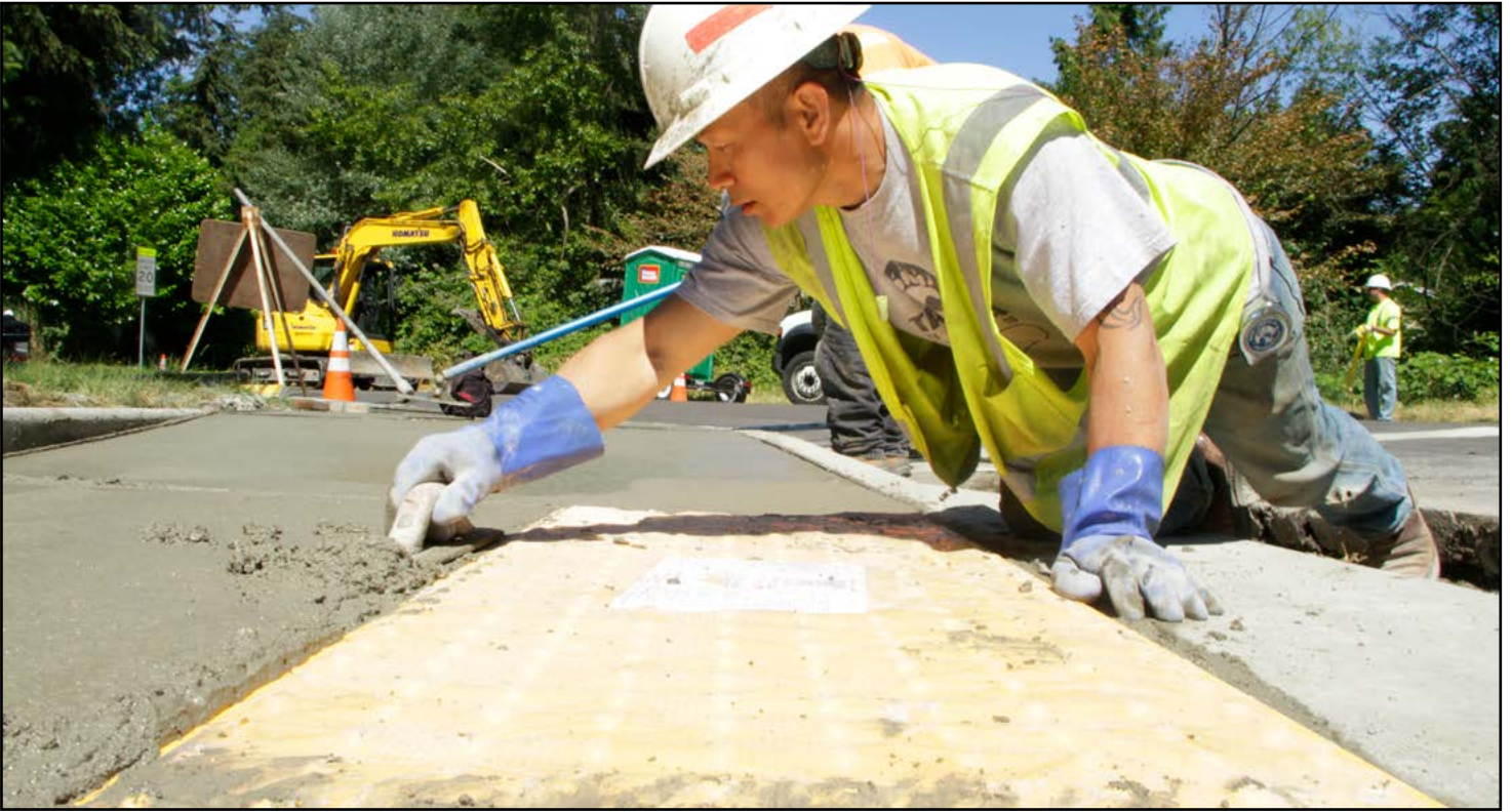
A contracted worker sculpts the concrete around the edges of a tactile warning strip along 100th Avenue Northeast, north of Northeast 125th Street. These tactile warning strips tell the vision-impaired they are about to enter a traffic zone.
