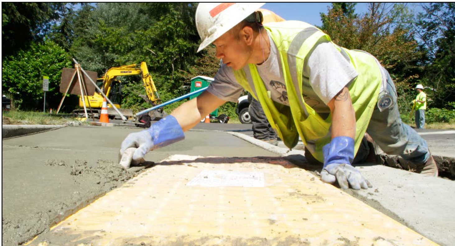
Westwater Construction worker Seth Phonpadith sculpts the concrete around the edges of a tactile warning strip along 100th Avenue Northeast, north of Northeast 125th Street. These tactile warning strips tell the vision-impaired they are about to enter a traffic zone.
