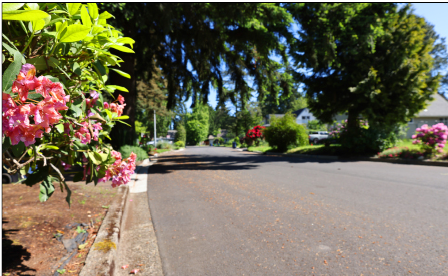
Kirkland's capital improvement program used levy funding in 2021 to repave 125th Avenue Northeast.
