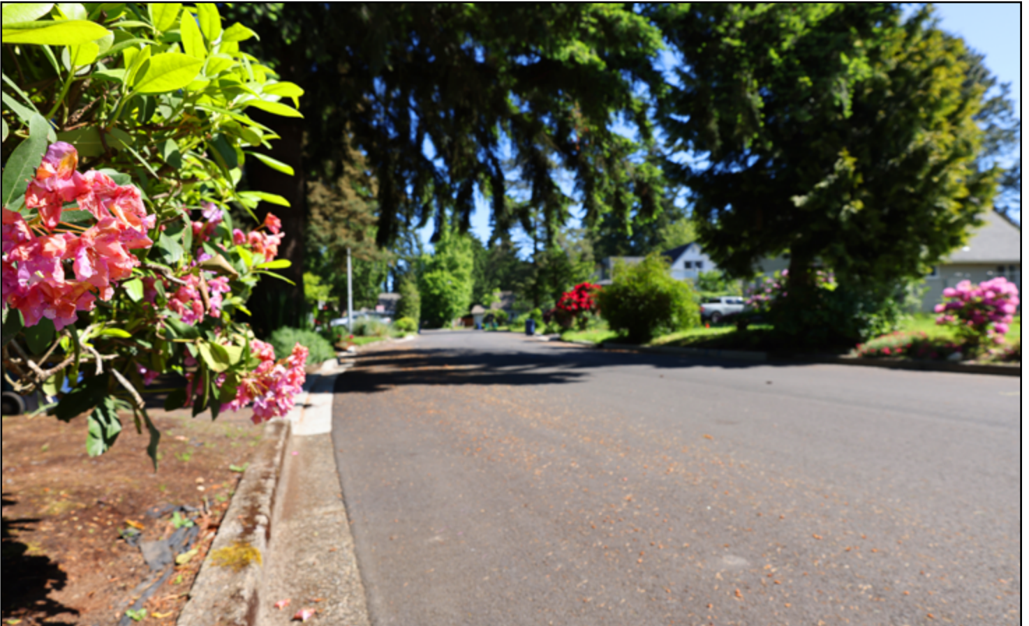
Kirkland's capital improvement program used levy funding in 2021 to repave 125th Avenue Northeast.
