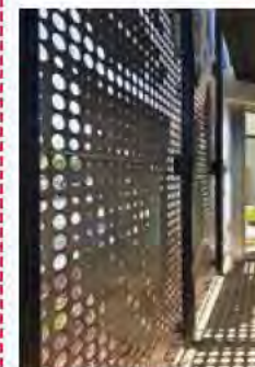
ALTERNATING PANELS WITH CIRCULAR PERFORATIONS RANGING IN SIZE FROM 1/2", 1", 1.5"
