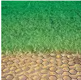
Turf Pavers @ Fire Lane
