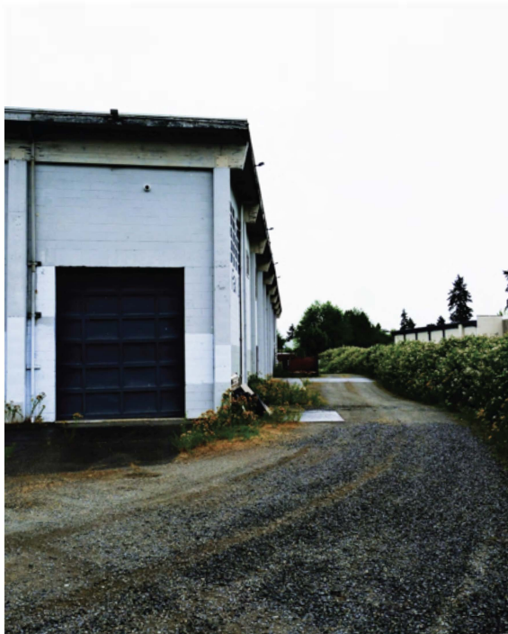
Potential Generator building
