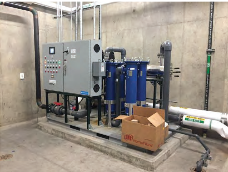
Figure 20 Part of onsite catchment water filtration system.
