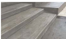
CAST IN PLACE CONCRETE STEPS
