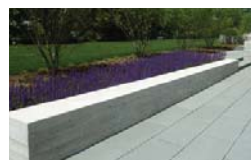
CAST IN PLACE CONCRETE SEATWALL
