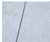
SANDBLASTED FINISH PAVING FIELD
