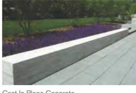
Cast In Place Concrete Seatwall
