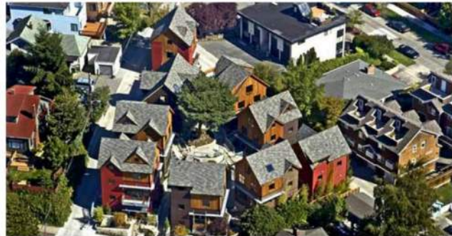
Detached, single-family homes in The Boulders at Green Lake development in Seattle, WA (images courtesy of Johnston Architects).
