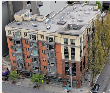
Cabrini Sr. Housing, First Hill 162 d/a, six story mixed use
