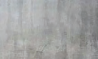
ARCHITECTURAL CONCRETE FINE / SACKED FINISH
