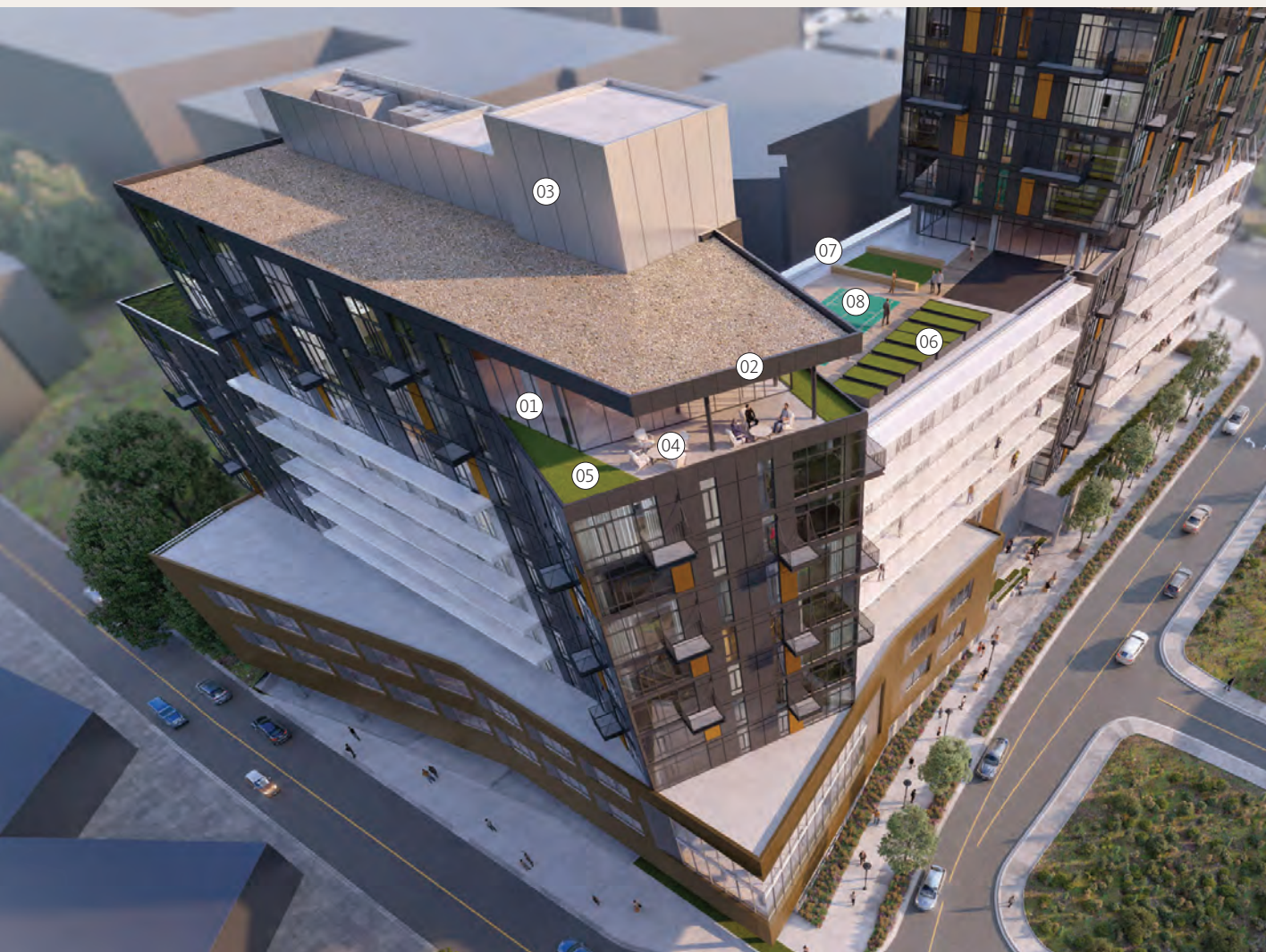
10 - South mass and scale // Rooftop facing Northwest
