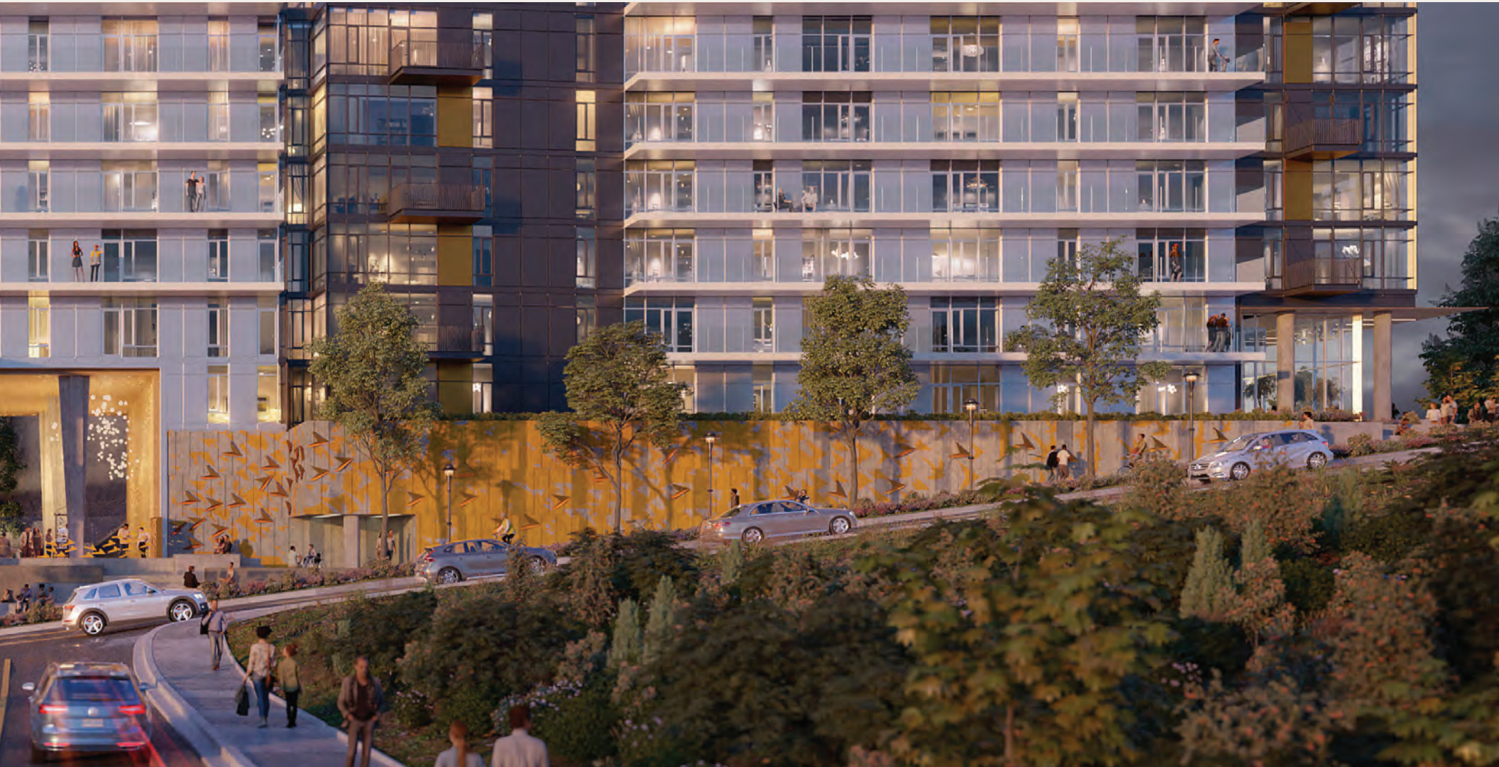
12 - 120th Avenue NE Facade
