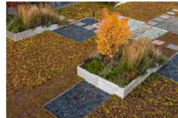
7 GREEN ROOF An area of green roof is provided on the terrace space between the public plaza and interior courtyard 'E'. The green roof is comprised of colorful tray plantings and raised planters with accent trees.
