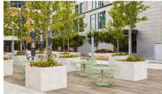
2 PUBLIC PLAZA The front entry space offers seating and short-term bike parking for building visitors and residents. Either side of the entry is generously landscaped to create a welcoming and obvious main entry into the building.
