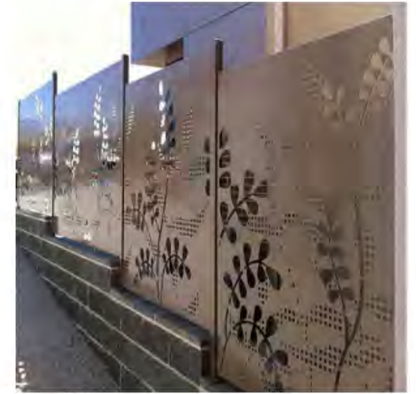
DECORATIVE METAL FENCE
