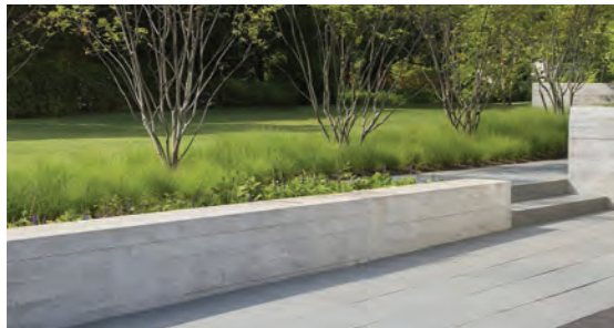
Board formed or special finish concrete planter walls in select public and private areas.
