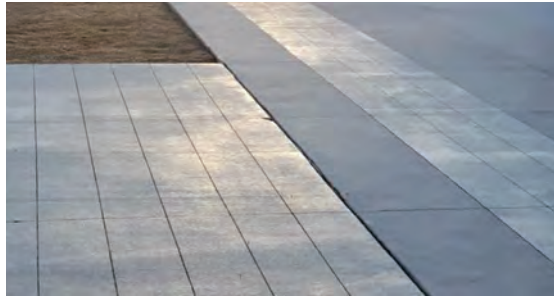
Cast-in-place concrete sidewalks with select areas of special finish such as integral color, special finish, or sawcut joints on the south through-block crossing.
