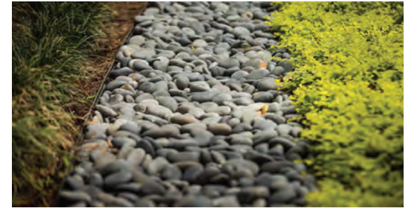
Metal edging to define areas with stone fill and planting over structure.
