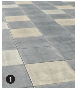
1 Existing precast pavers
