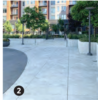
2 Existing PIP concrete
