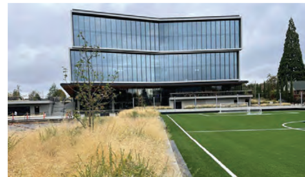
Recently planted 2' - 3' depth
