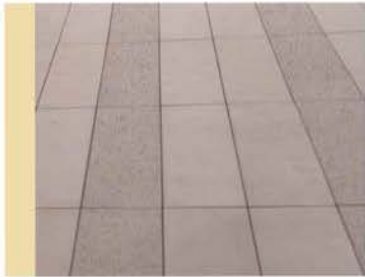
2' bands with heavy etched finish
