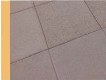
2' Scoring with medium etched finish, square pattern 2x2
