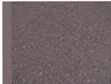
Exposed aggregate finish
