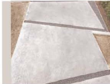
Exposed aggregate concrete band pattern
