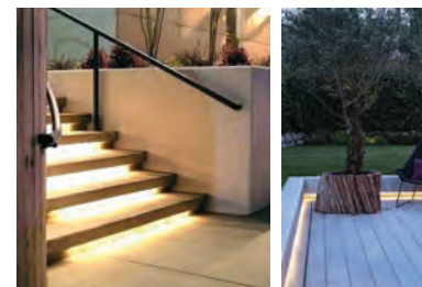
ACCENT LIGHTING AT COURTYARD PLAZA
