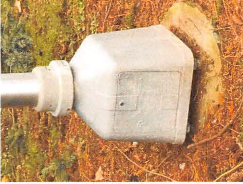
Pole close up
