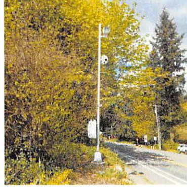
Pole close up
