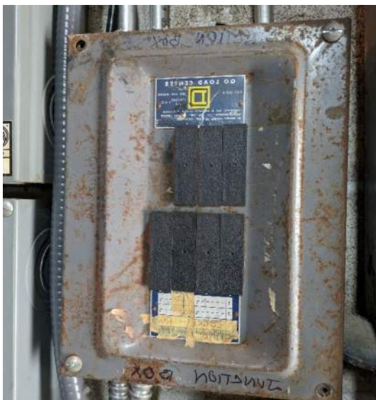
Photo 7- Assumed ACM 6"x8" Junction box Storage
