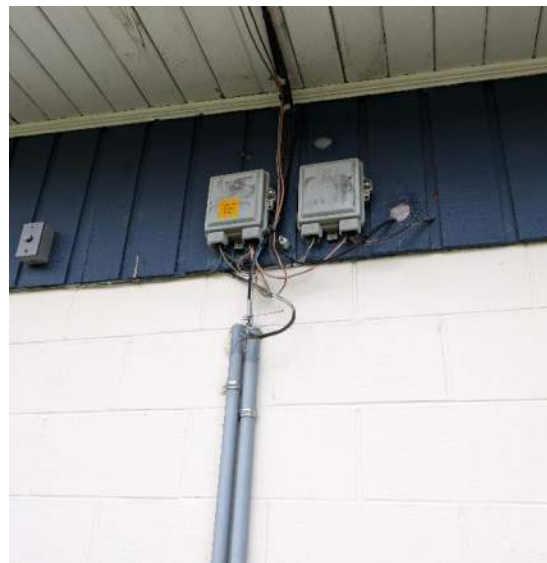
Photo 8 – Telephone network interface Exterior side of Storage Exterior blue and white paint on wood soffit and CMU
