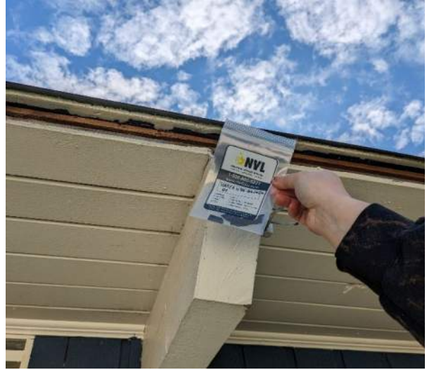
Photo 2- Sample 11711-050724-01 (Fiberglass paneling) over asphalt shingles on Assumed ACM Vapor Barrier (on wood sheathing) Roof Result: ND (all layers)
