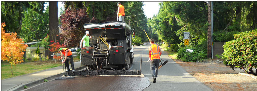
City of Kirkland road crew applying Slurry Seal..
