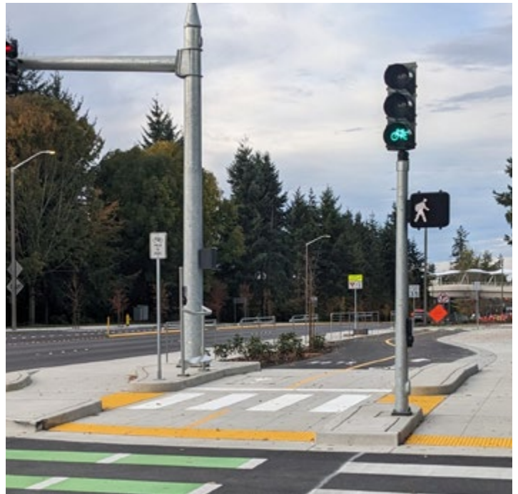
Figure 67. Bicycle Signal Head in Redmond, WA
