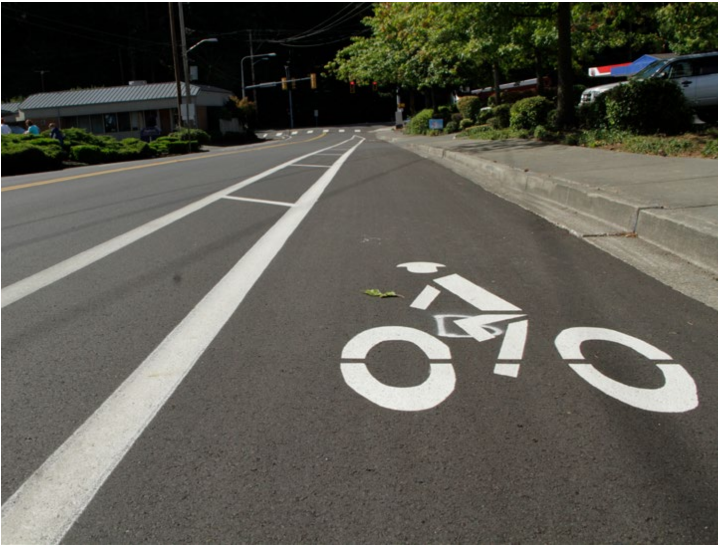
Figure 20. Buffered bicycle lane on NE 141st St
