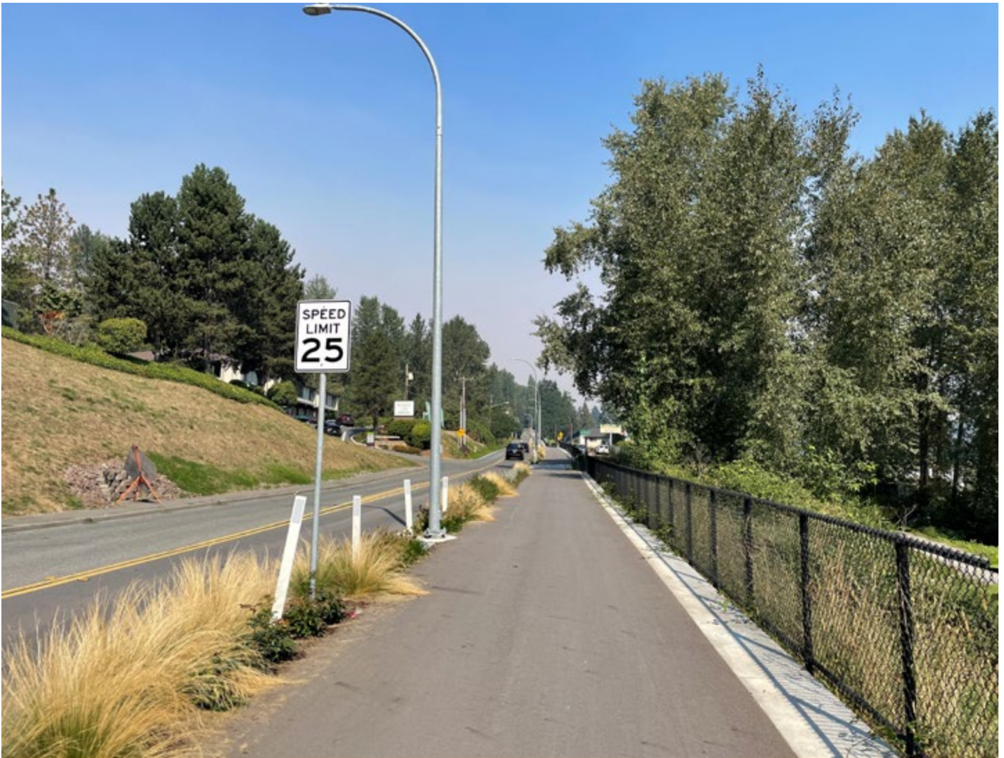
Figure 39. Willows Road NE shared-use side path
