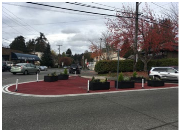
Figure 54. Paint and Post Curb Extension with Planters in Seattle, WA
