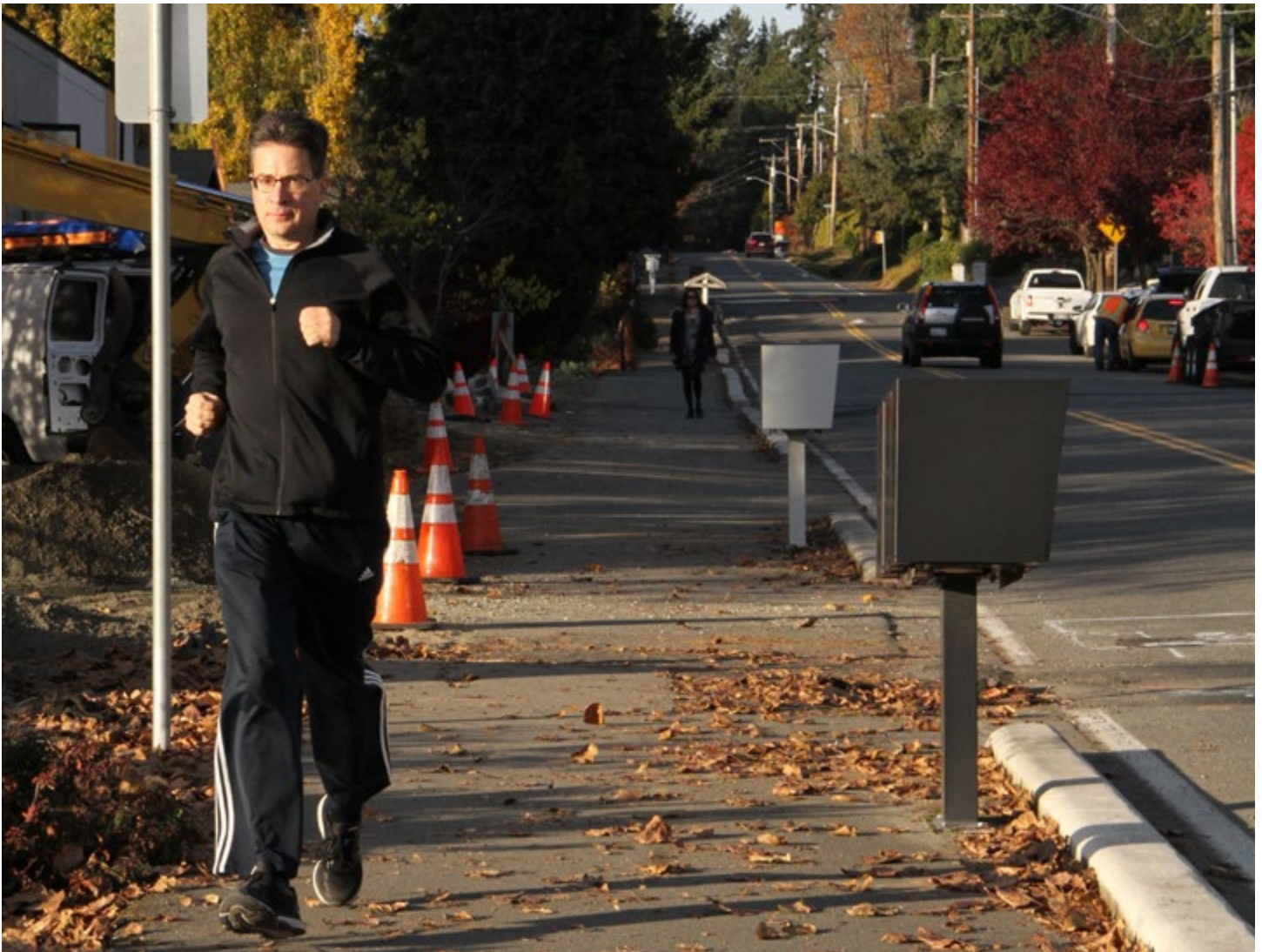
Figure 7. On-street temporary walkway on 112th Ave NE
