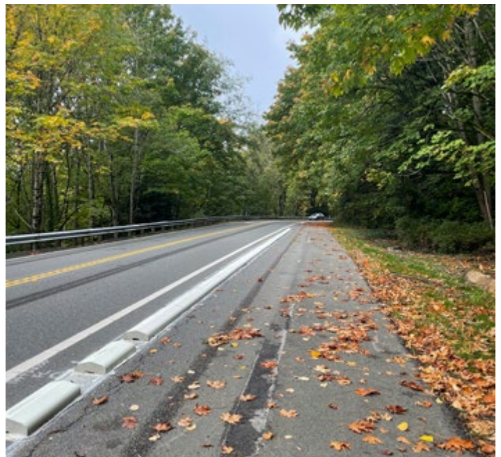
Figure 9. Walkway with Extruded Curbs on 90th Ave NE
