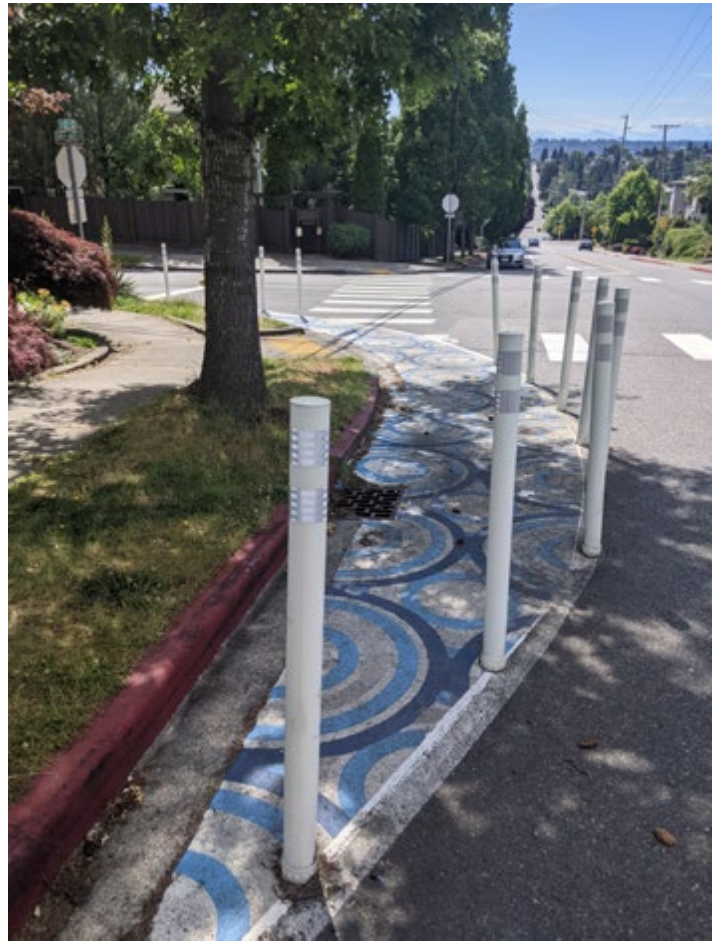
Figure 53. Paint and Post Curb Extension on NE 87th St and 114th Ave NE
