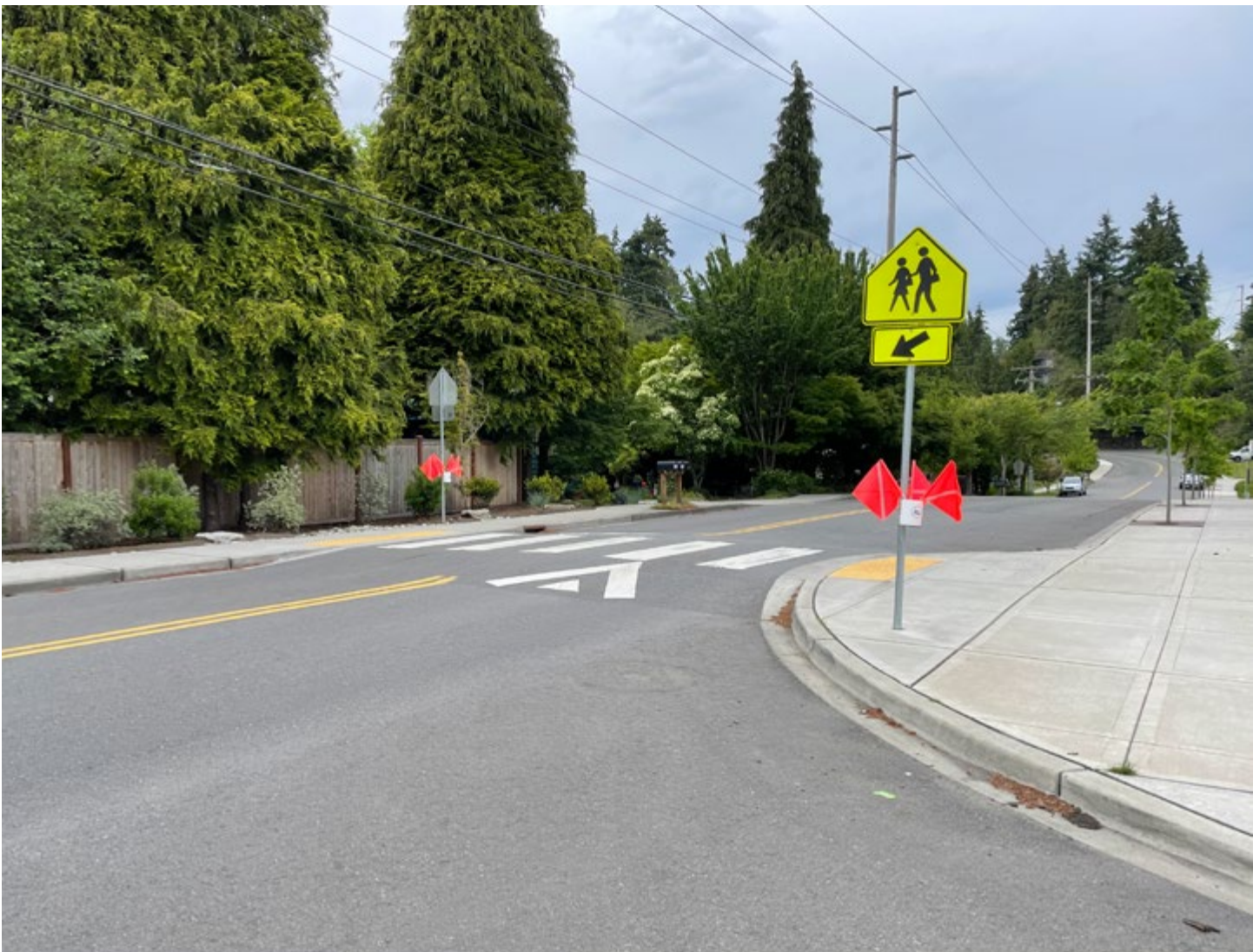
Figure 47. Raised crossing on 6th St at Peter Kirk Elementary
