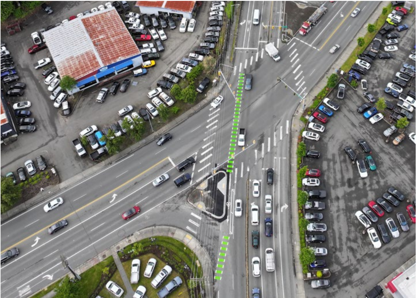
Figure 68. Green Conflict Markings through the intersection of NE 124th St and Slater Ave NE
