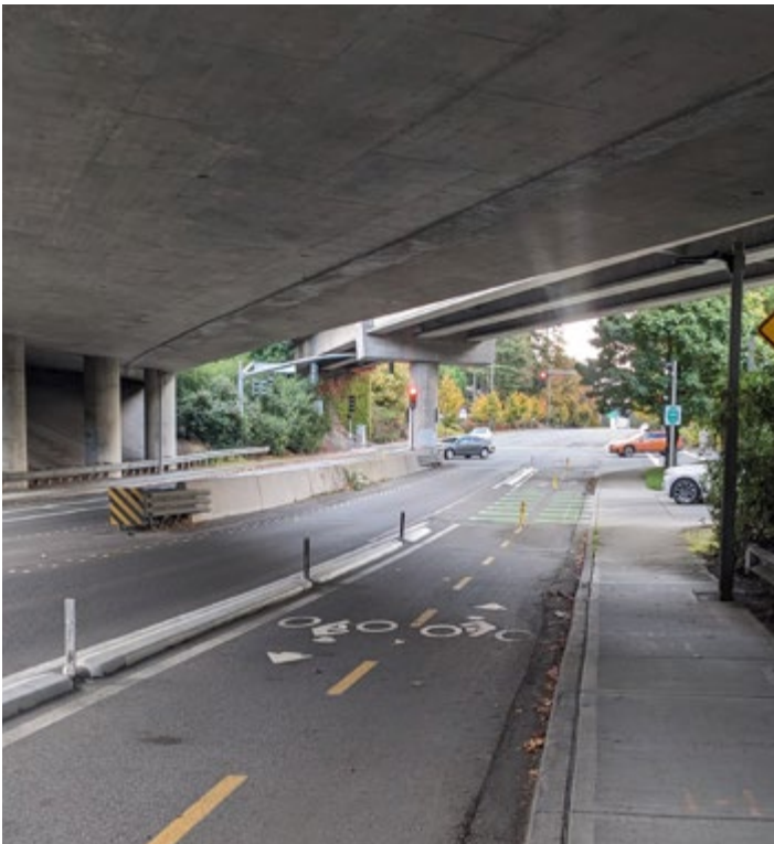
Figure 31. Quick build street-level protected bicycle lanes with extruded curb and flex posts in Bellevue, WA
