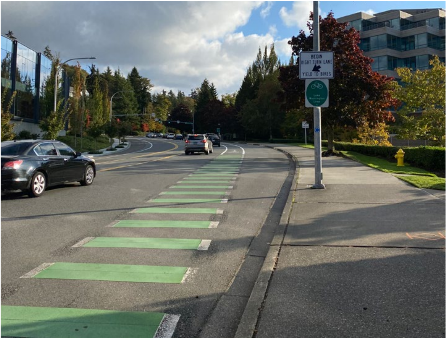
Figure 81. Bike lane at added right turn lane transition on Lake Washington Blvd NE
