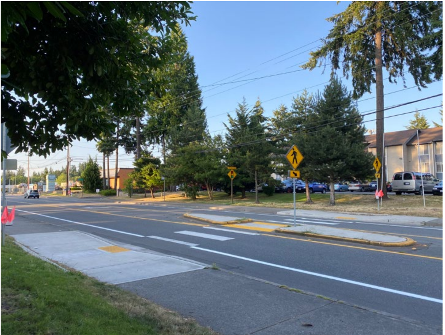
Figure 55. Median island on 124th Ave NE near the Kingsgate Library
