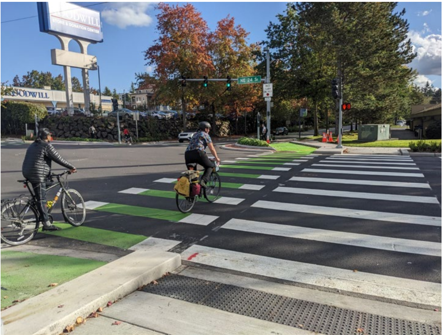
Figure 78. Protected intersection at 152nd Ave NE and NE 24th St in Redmond, WA
