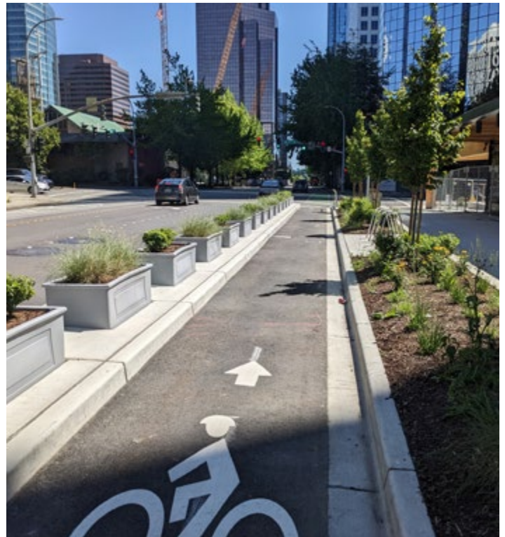
Figure 32. Permanent street-level protected bicycle lane with concrete median islands and planter boxes in Bellevue, WA
