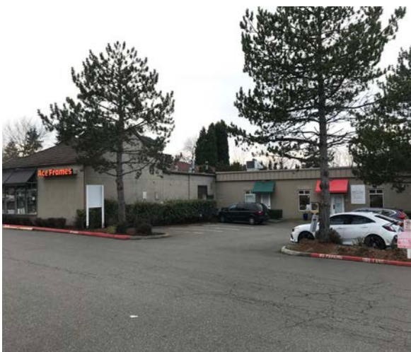
Photo 5 Bldg. 2 rear portion
