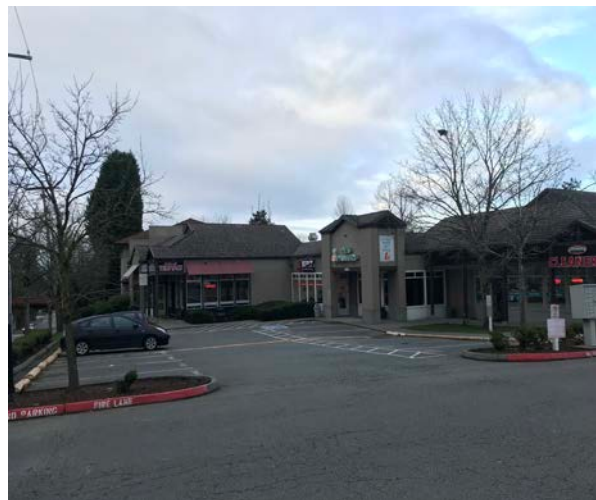
Photo 4 Front of Building 2
