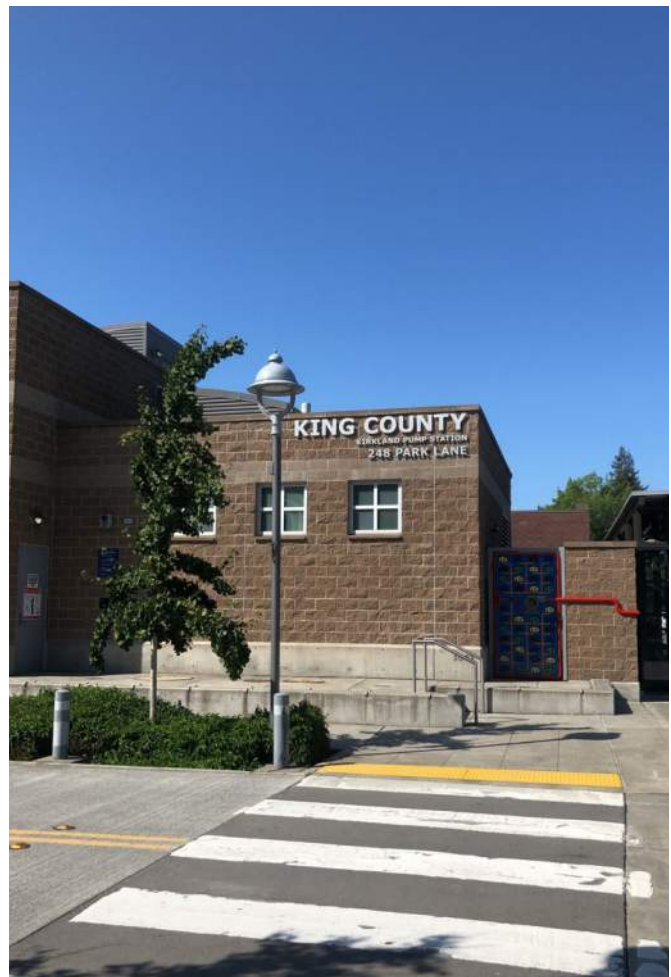
Pump Station in Downtown Kirkland
