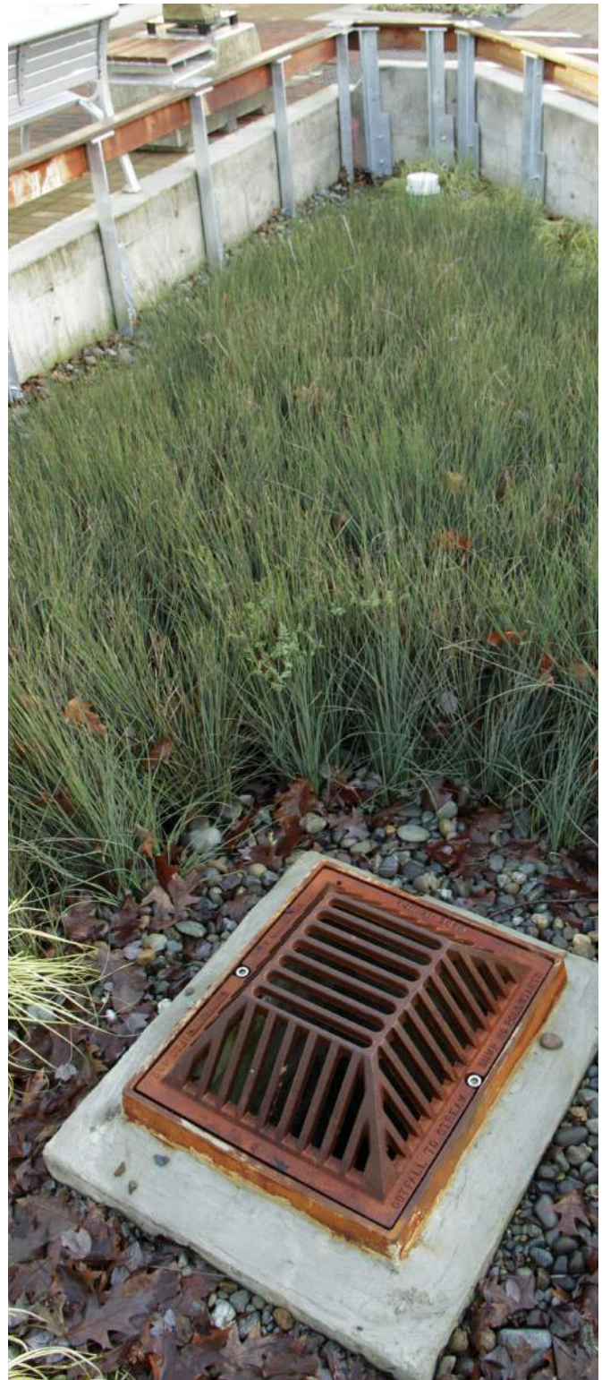
Bio retention in Park Lane
