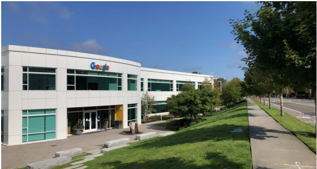
Google Campus along 6th Street
