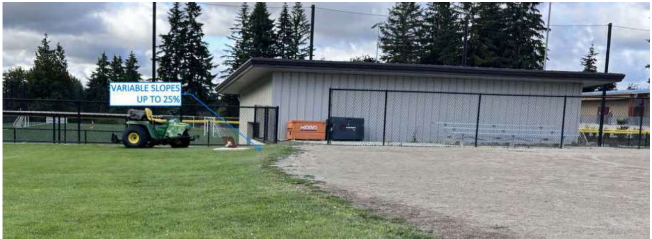
Image 4, 3 rd Base Line / Foul Territory Grade Irregularities
