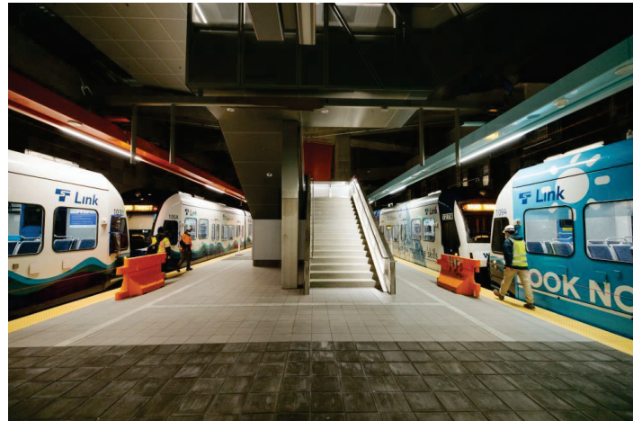
Test trains at U District Station
