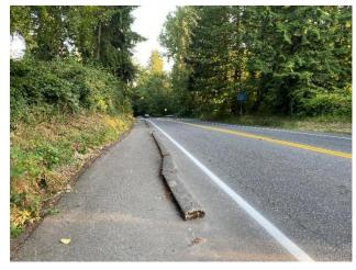
King County installed sections of extruded curb along the north side of 90th Avenue NE/131st Way as a form of surface water control. The original purpose of the curb was to stop surface water run-off from entering the roadway where it would sheet-flow across to the other side and occasionally freeze in winter months. The curb is now broken in many places and no longer functions as intended. The broken extruded curb also presents a hazard for people walking, biking and driving in the corridor.
