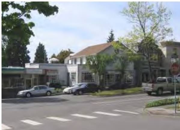
Office buildings on Market Street
