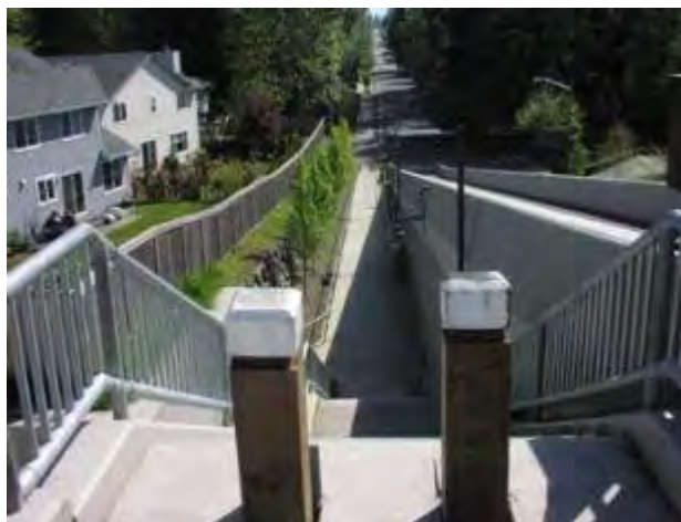
The existing Emergency and Nonmotorized Overpass at NE 100th Street provides a connection between Highlands and the North Rose Hill neighborhood.
