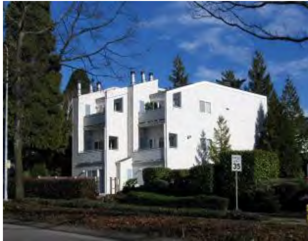
Multi-family Development on Market Street
