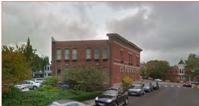
Sears Building at 701 Market Street
