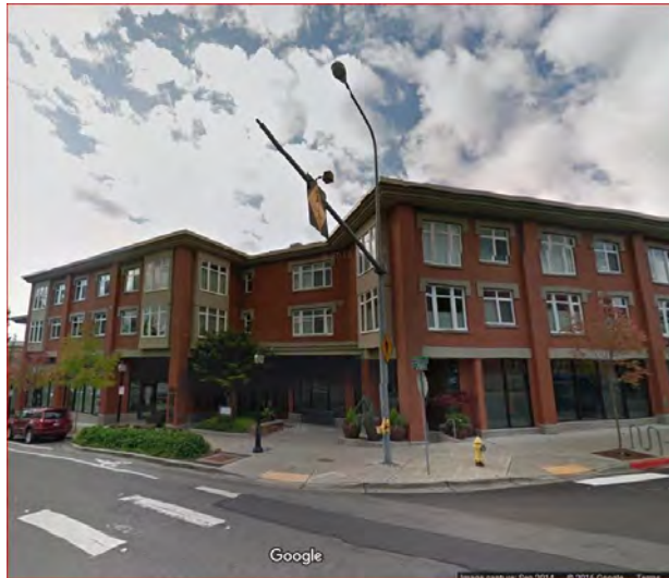
Intersection at 7th Avenue and Market Street
