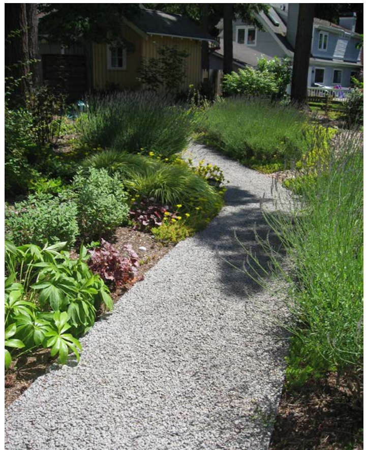
Pervious paving at a development in Kirkland.
