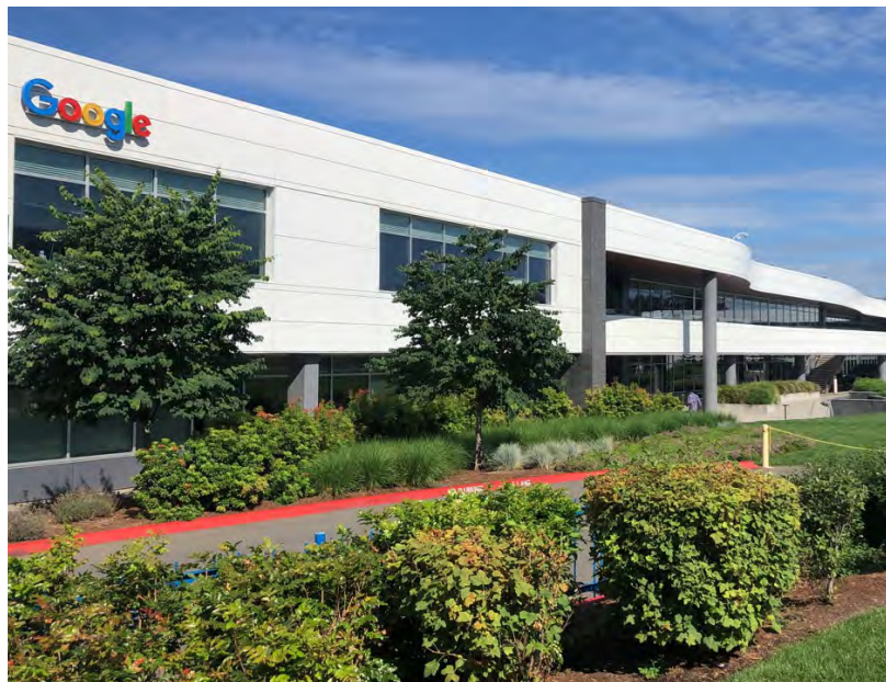
Kirkland's Google campus was built to be resource efficient, targeting LEED Platinum standards.
