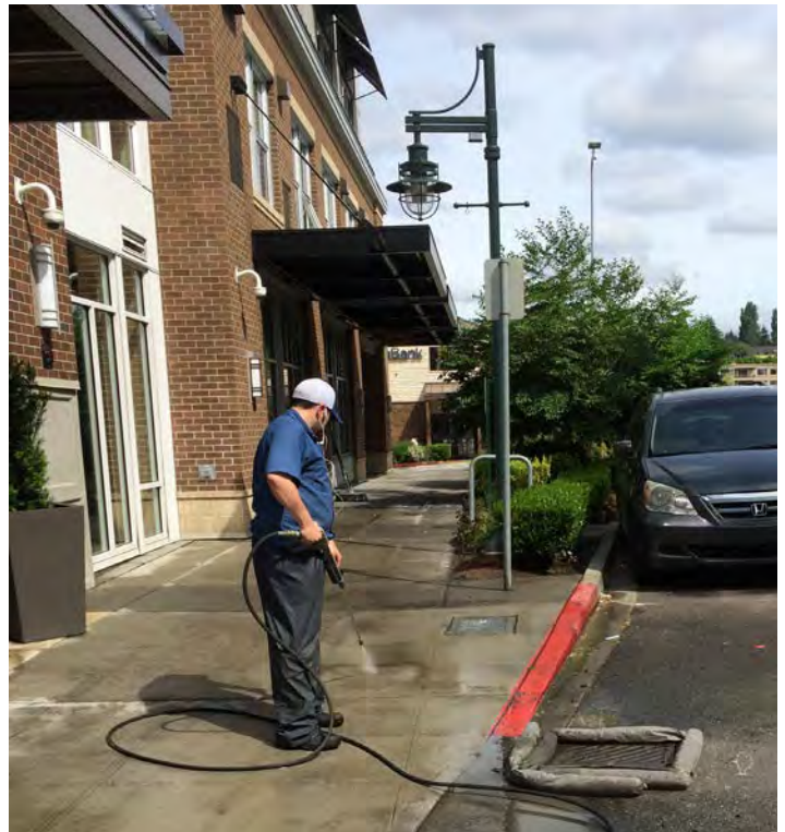
Pressure washing with an absorbent sock around the storm drain protects our water from pollution.
