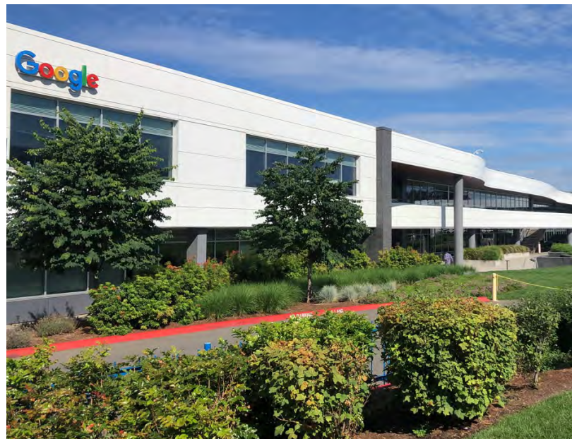
Kirkland's Google campus was built to be resource efficient, targeting LEED Platinum standards.
