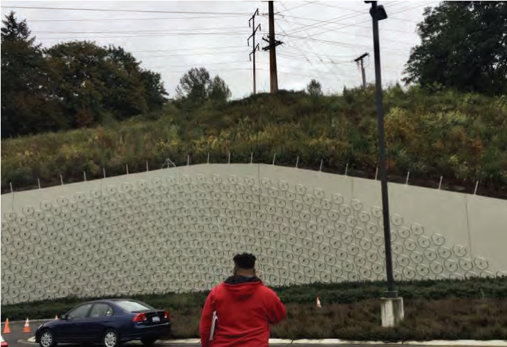
Figure 22 Retention wall and art installation of reflecting circles.
