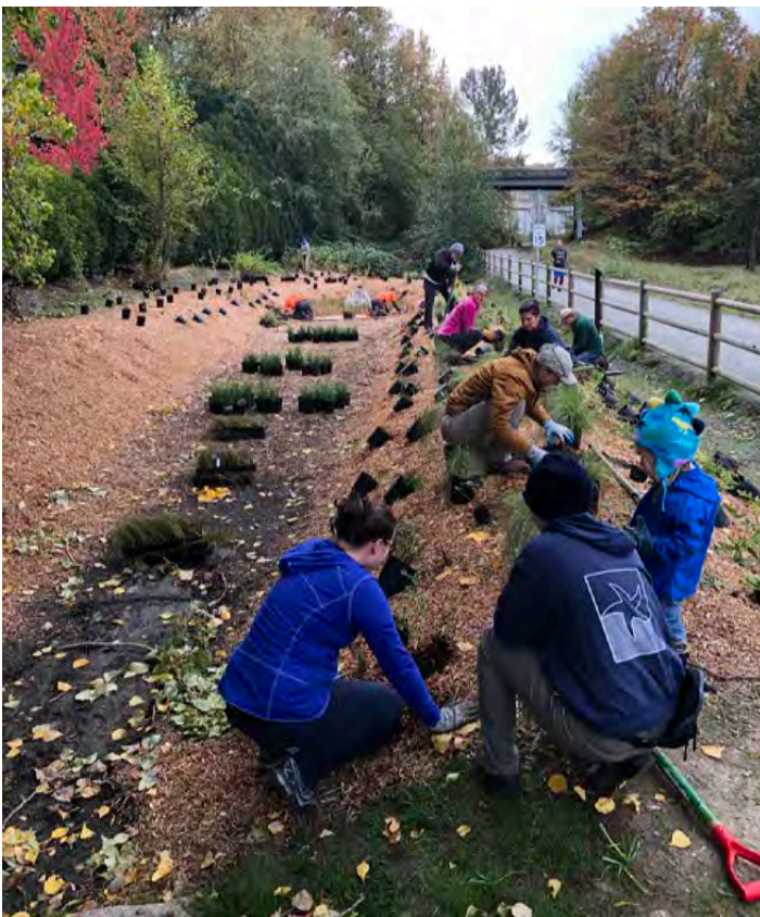
Volunteers from a Kirkland business and other community members plant native plants at a newly-constructed rain garden along the Cross Kirkland Corridor in the Highlands neighborhood.
