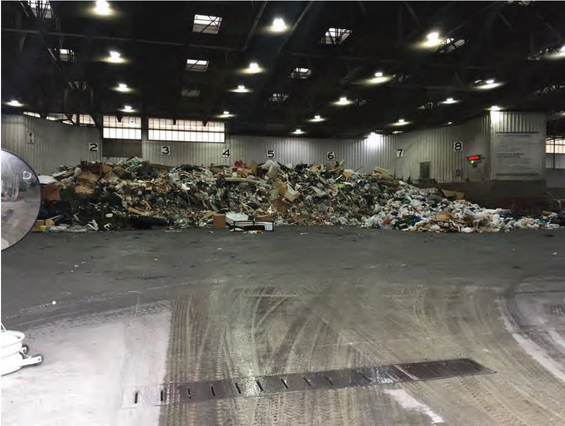
Figure 12 Commercial waste drop-off truck entrance.
