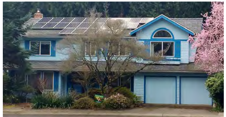
Solar panels installed at a Kirkland home during a Solarize Kirkland campaign.
