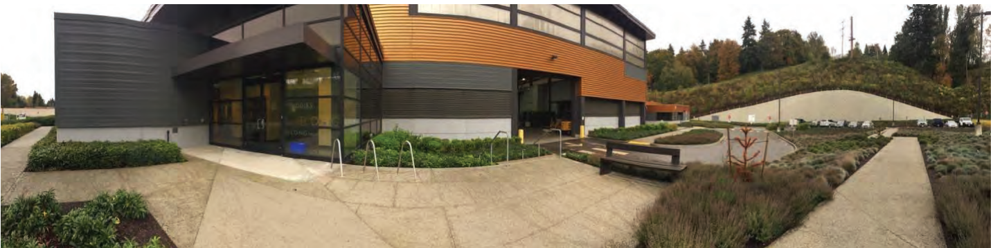
Figure 4 Panoramic view (distorted) of front door entrance portico extending to visitor parking and retainer wall.
