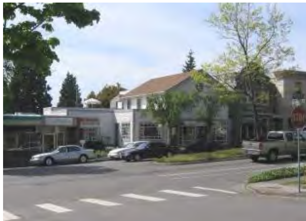
Office buildings on Market Street
