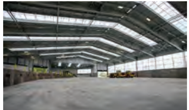
Skylights and translucent windows at Bow Lake Recycling and Transfer Station
