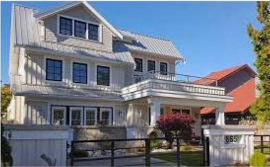
Kirkland, WA | State Roofing | Roofing ...
