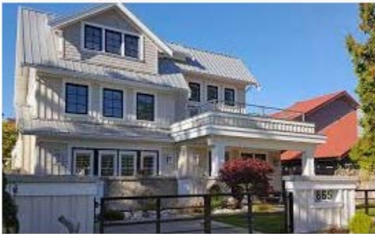
Kirkland, WA | State Roofing | Roofing ...
