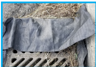
Untrimmed filter fabric creates flooding.
