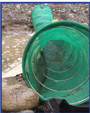
Reusable check dams such as Spring Berms can be very cost effective over time and are easy to install.
