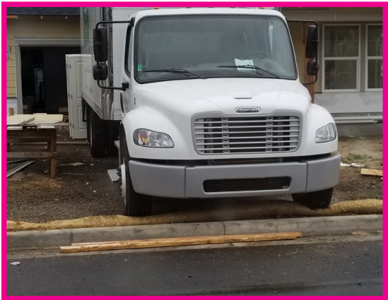
Perimeter controls can be easily damaged and must be monitored and replaced as necessary by onsite personnel.
