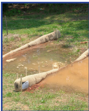
Fiber rolls such as TerraTube can filter the water as well as slow velocity.
