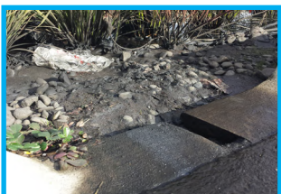
Sedimentation of bioretention facilities may require replacement of the media and plantings.
