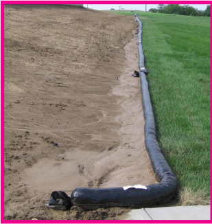
Durable and reuseable wattle that can go from project to project.
