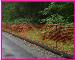
Perimeter control with filtration using a compost sock.
