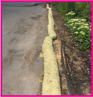
Stormwater will easily undercut wattles that are not trenched in, not staked, and not overlapped appropriately.
