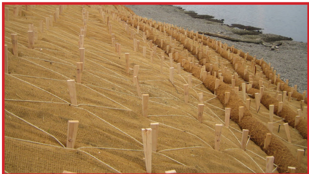
Slope checks and covering BMPs used in combination are effective for erosion prevention and seed establishment
