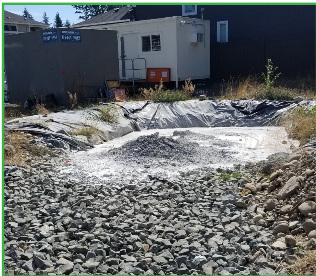
Concrete washout pits can be created on site with a liner; however, the water and solids in the pit must be properly disposed of.
