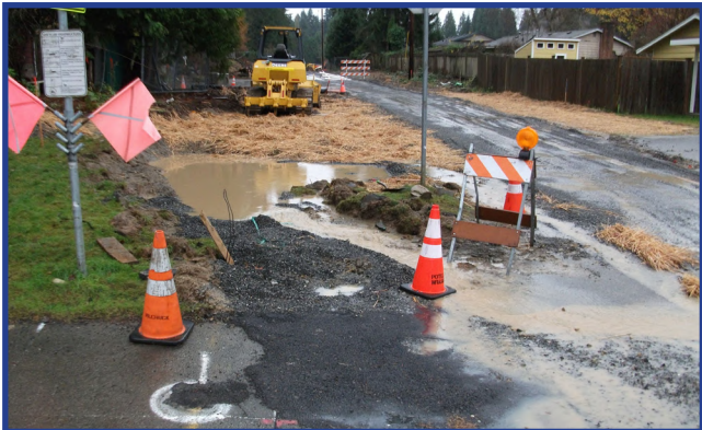
Insufficiently sized and maintained sediment trap .
