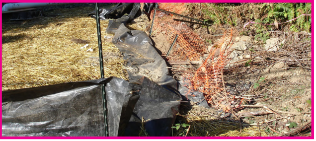
Sediment fence without wire backing is easily brought down by wind or water. Only wire backed sediment fence is allowed in Kirkland.
