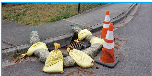
In some situations, above-grate protection in addition to the filter can make the inlets more maintainable.
