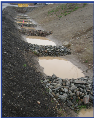
Check dams slow the flow of water and allow sediment and debris to drop out.
