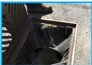
Trim extra filter flap or use an adjustable metal framed insert.
