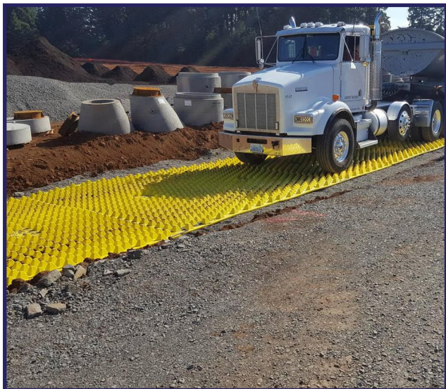
An example of heavy duty plastic plates that are adaptable and reusable for construction entrances.
