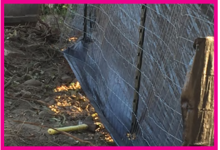
Wire backed sediment fence that is not keyed in is ineffective.
