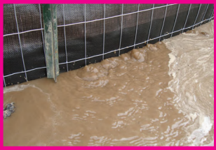
Undercutting of the wire backed sediment fence can occur if not trenched in and happens most frequently near the stake.
