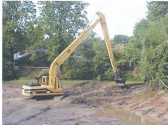
Figure 1.14: Muck removal and slope dressing by long reach backhoe
