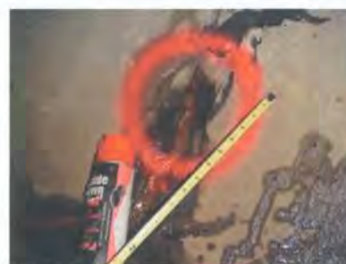
Figure 5.8: Rust intrusion demonstrates improper pipe joint.
