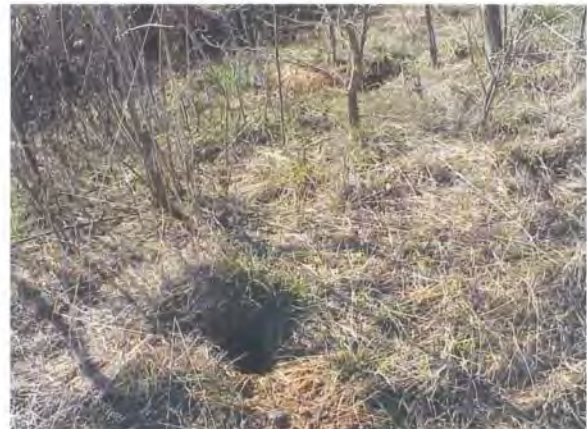
Figure 1.20: Animal burrow in pond embankment.
