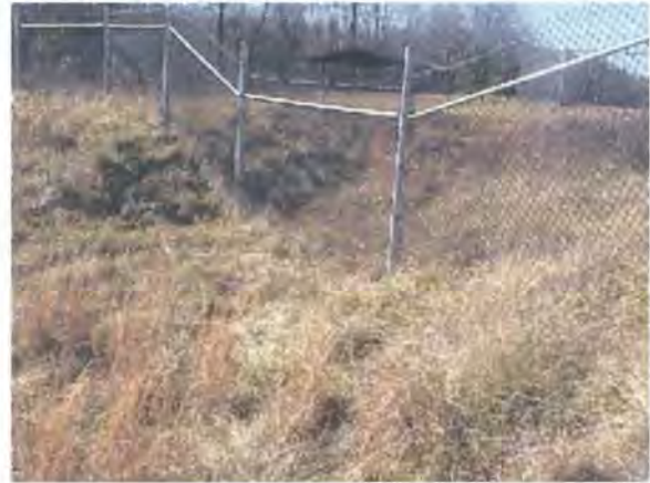
Figure 2.1: Fence across Emergency Spillway
