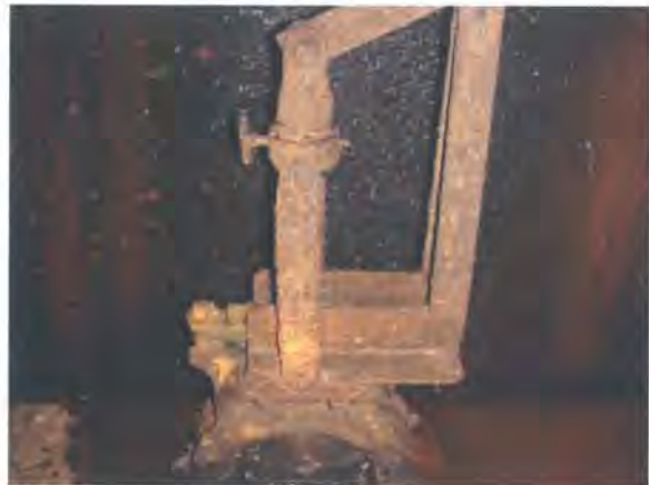
Figure 1.19: Corroded plumbing and valve.
