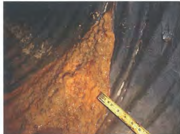
Figure 5.6: Soil entering open pipe joint.
