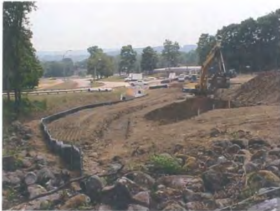
Figure 3.2: Dam construction - Photo 1
