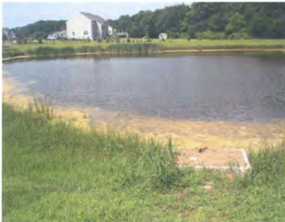
Figure 1.5: Flattop riser covered with debris.
