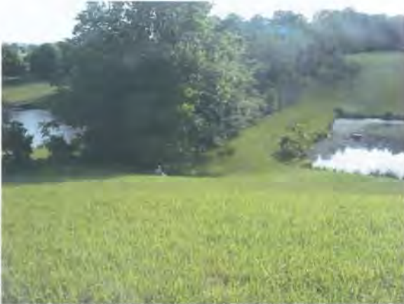
Figure 1.11: Woody vegetation on embankment
