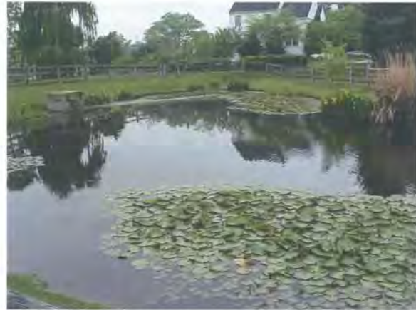
Figure 2.4: Riser located near pool edge for easier access.
