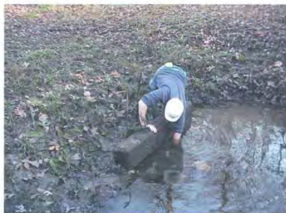
Figure 5.3: Clogged low flow orifice (before maintenance)
