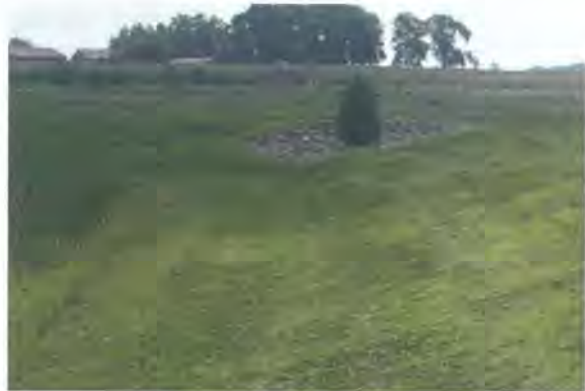
Figure 5.14: Unwanted vegetation - tree on embankment
