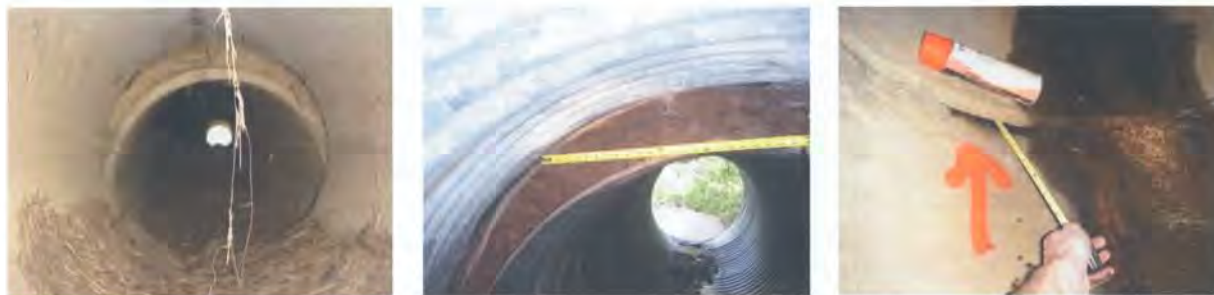
Figure 5.7: Misalignment in RCP (left and right) and CSP (center) applications.
