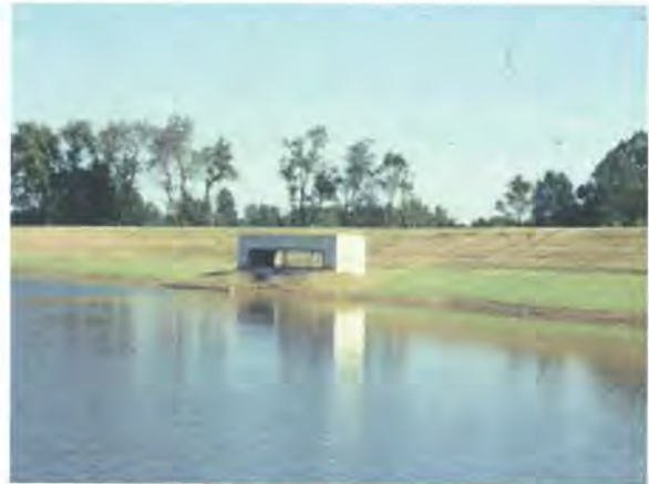
Figure 5.1: Riser located near pool edge for easier access.
