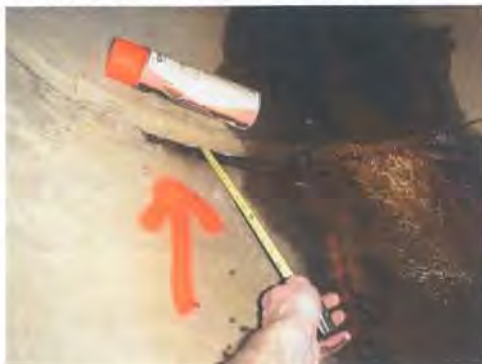
Figure 4.3: Marking pipe joint separation
