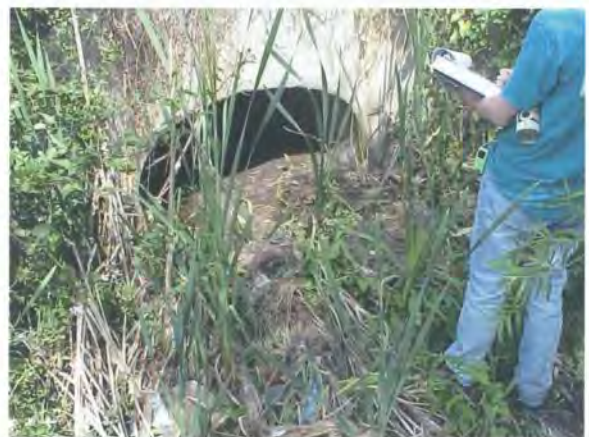
Figure 5.11: Excessive vegetation near an outfall
