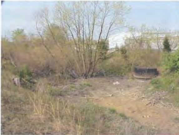
Figure 1.13: Sediment accumulation in a dry pond
