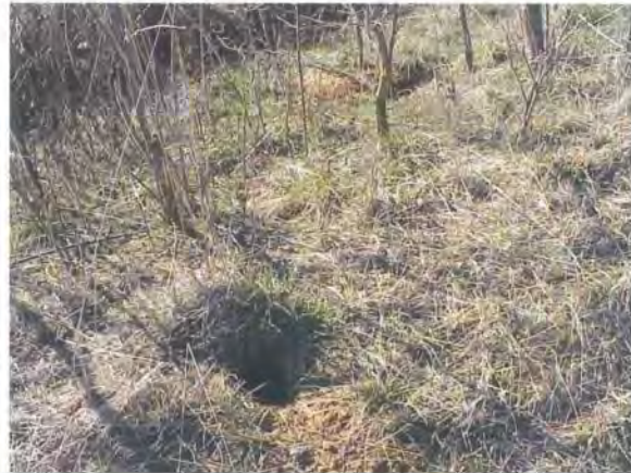
Figure 5.27: Animal burrow in pond embankment.
