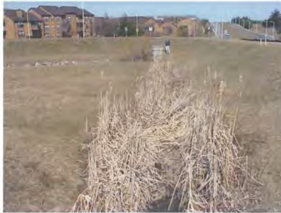
Figure 5.15: Vegetation establishment where the inflow channel slope is inadequate to drain properly.
