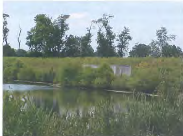
Figure 1.12: Excessive vegetative growth obscures riser
