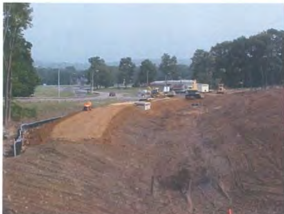
Figure 3.4 Dam construction – Photo 3
