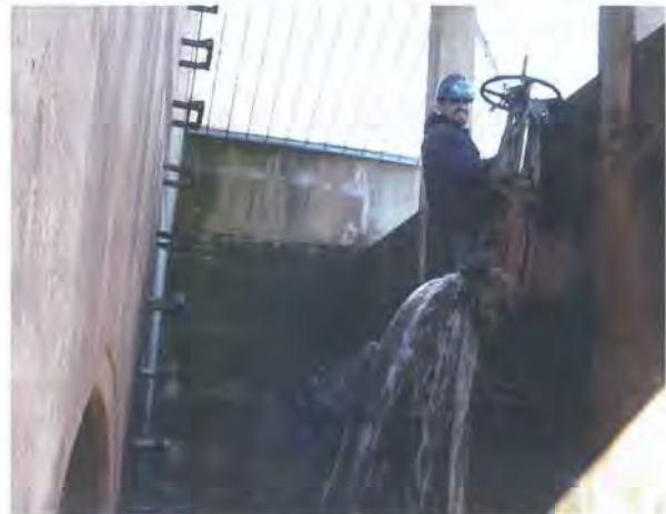
Figure 5.2: Clogged valve
