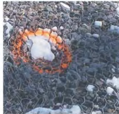
Figure 4.4: Marking a hole in gabion fabric
