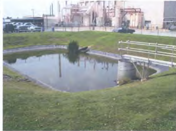
Figure 1.6: Riser without trash rack
