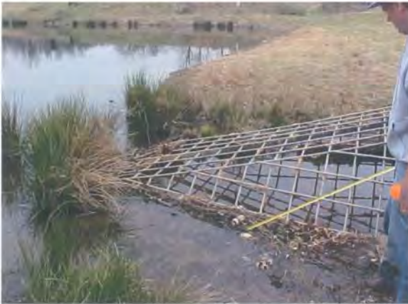
Figure 1.4: Abnormally high permanent pool – Water spills into 2- year weir because beavers have clogged the low flow orifice.
