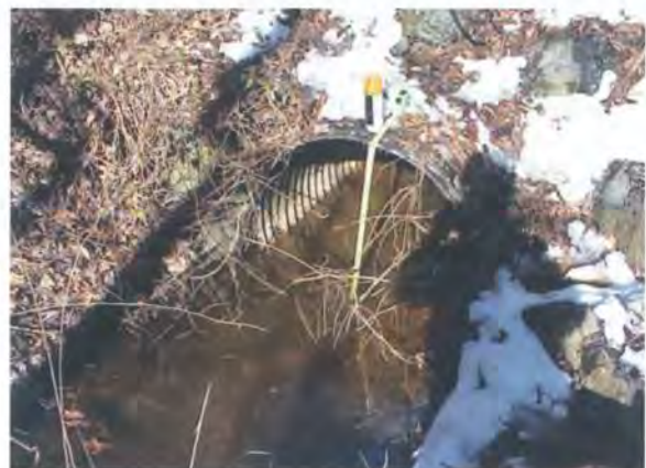
Figure 5.22: Forced access location.
