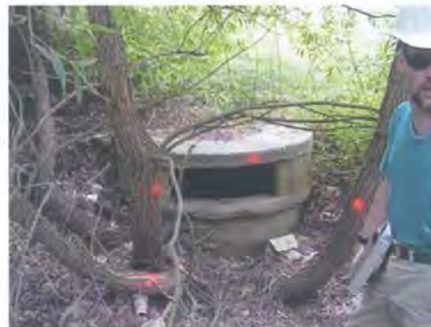
Figure 4.2: Marking trees to be removed.
