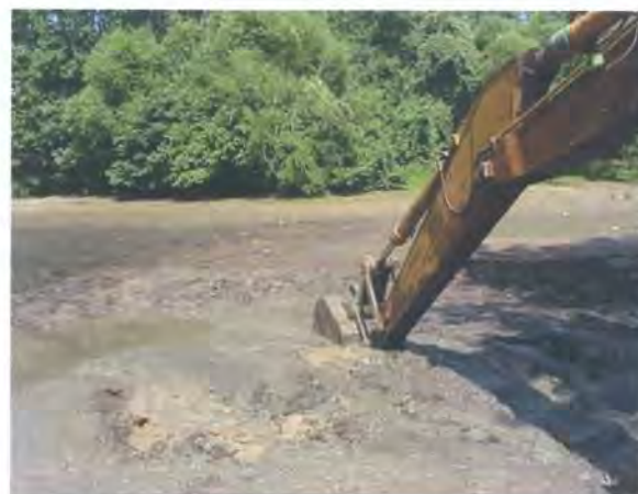
Figure 5.19: Mechanical dredging with backhoe.
