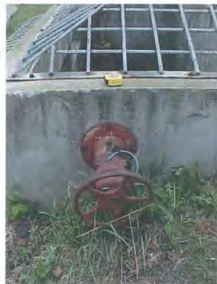
Figure 5.25: Valve outside riser.
