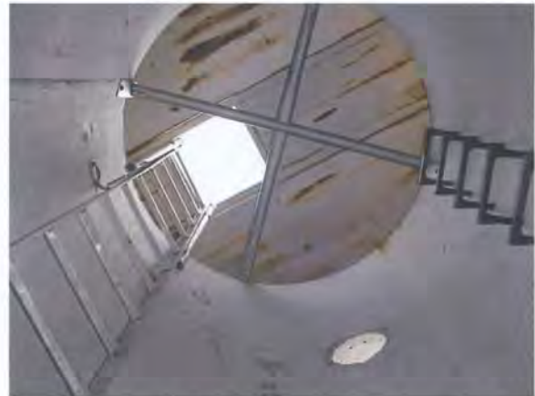
Figure 1.16: Ladder and steps in riser.
