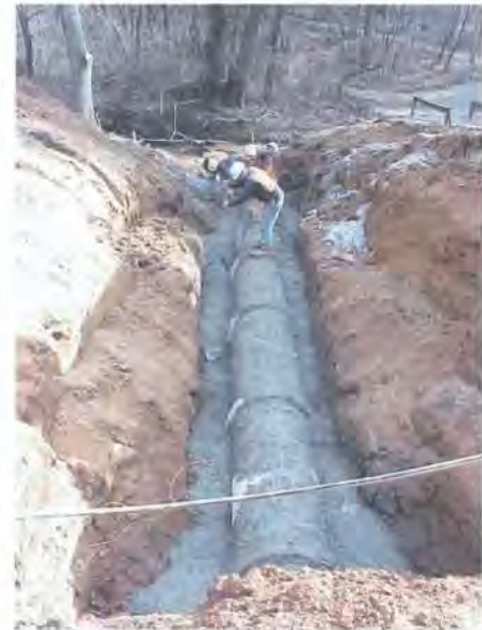
Figure 3.1: Barrel laid in concrete cradle
