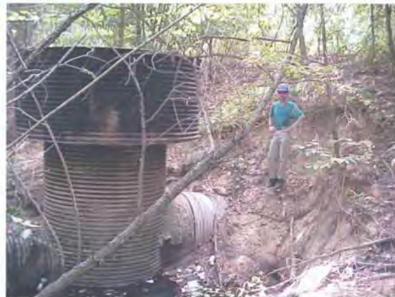
Figure 1.8: Severe erosion around riser and barrel
