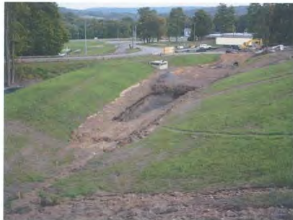
Figure 3.5 Dam construction – Photo 4
