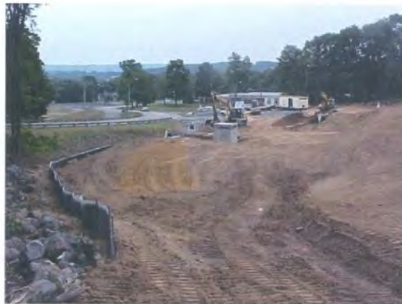
Figure 3.3 Dam construction – Photo 2
