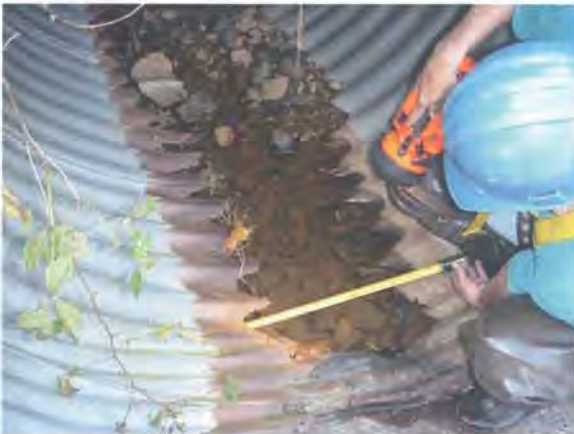
Figure 1.7: Pipe invert abrasion
