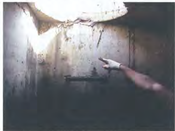
Figure 5.21: Missing manhole step
