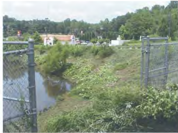
Figure 2.6: Chain link fence
