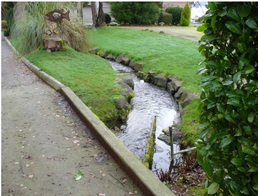
Photo #2. Holmes Point Creek confined to constructed channel
