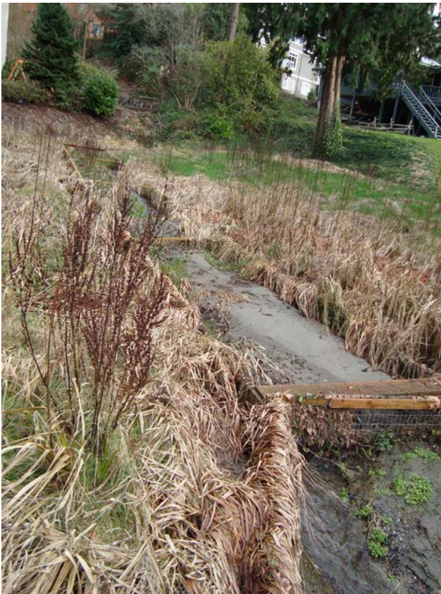
Photo #4 Channel upstream of dam filled with sediment and reed canary grass
