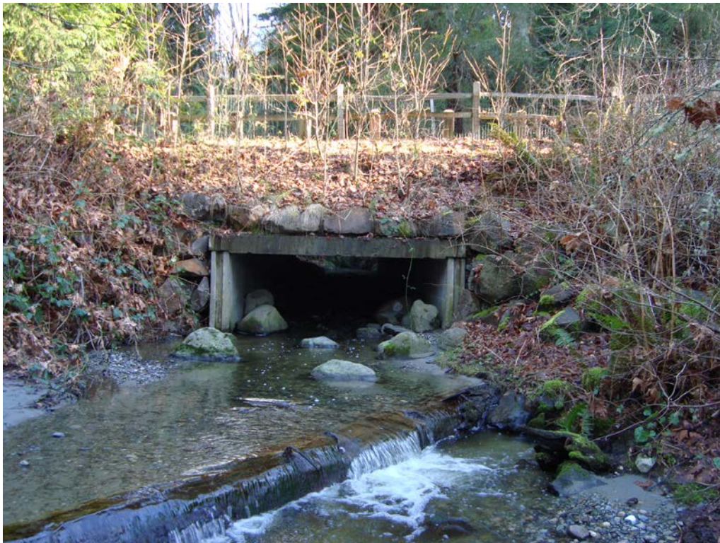
Photo #4. Holmes Point Drive 10-ft wide box culvert looking upstream
