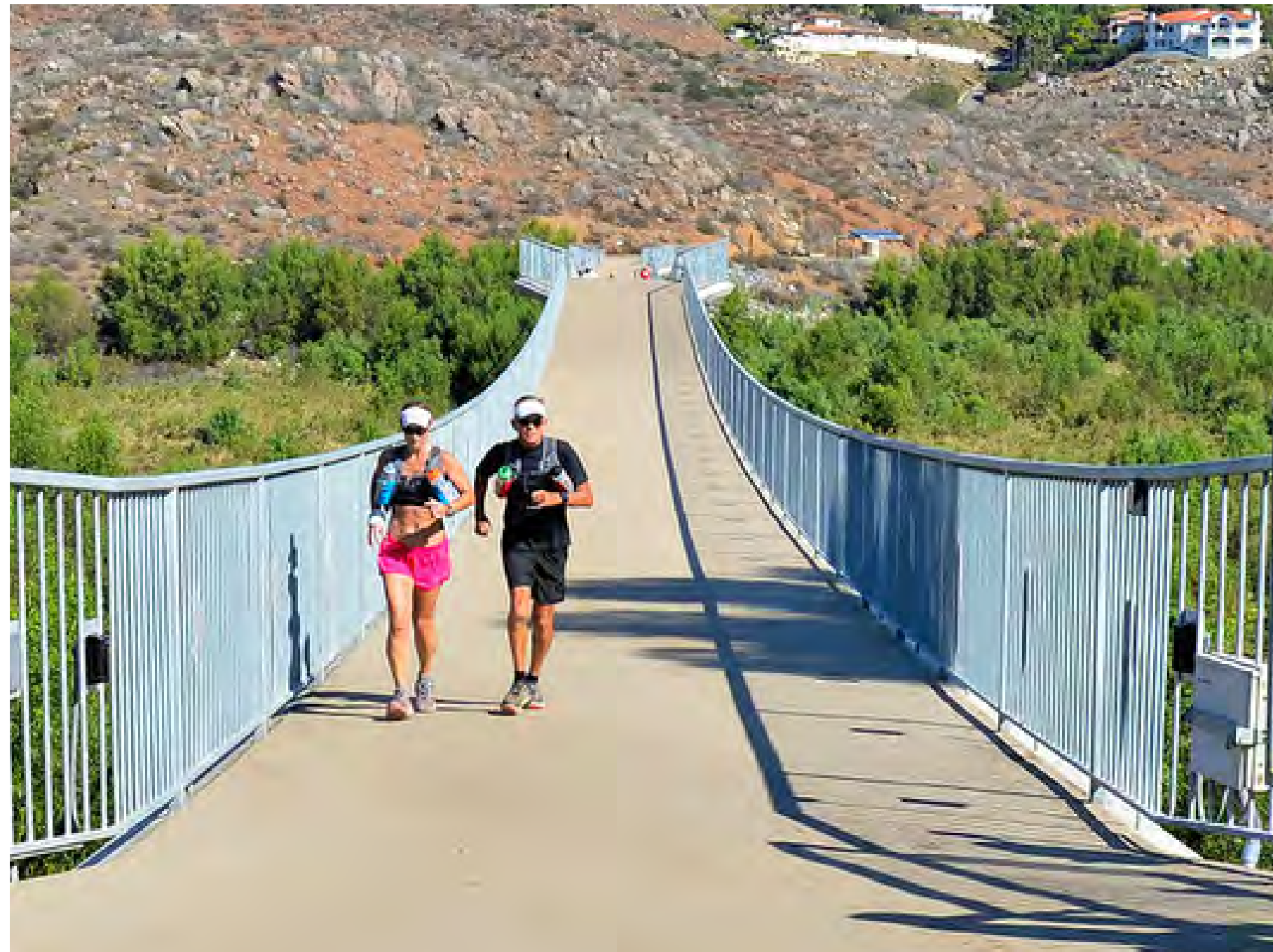
LAKE HODGES PEDESTRIAN BRIDGE STRESS RIBBON 12 FOOT CLEAR WIDTH SAN DIEGO, CA
