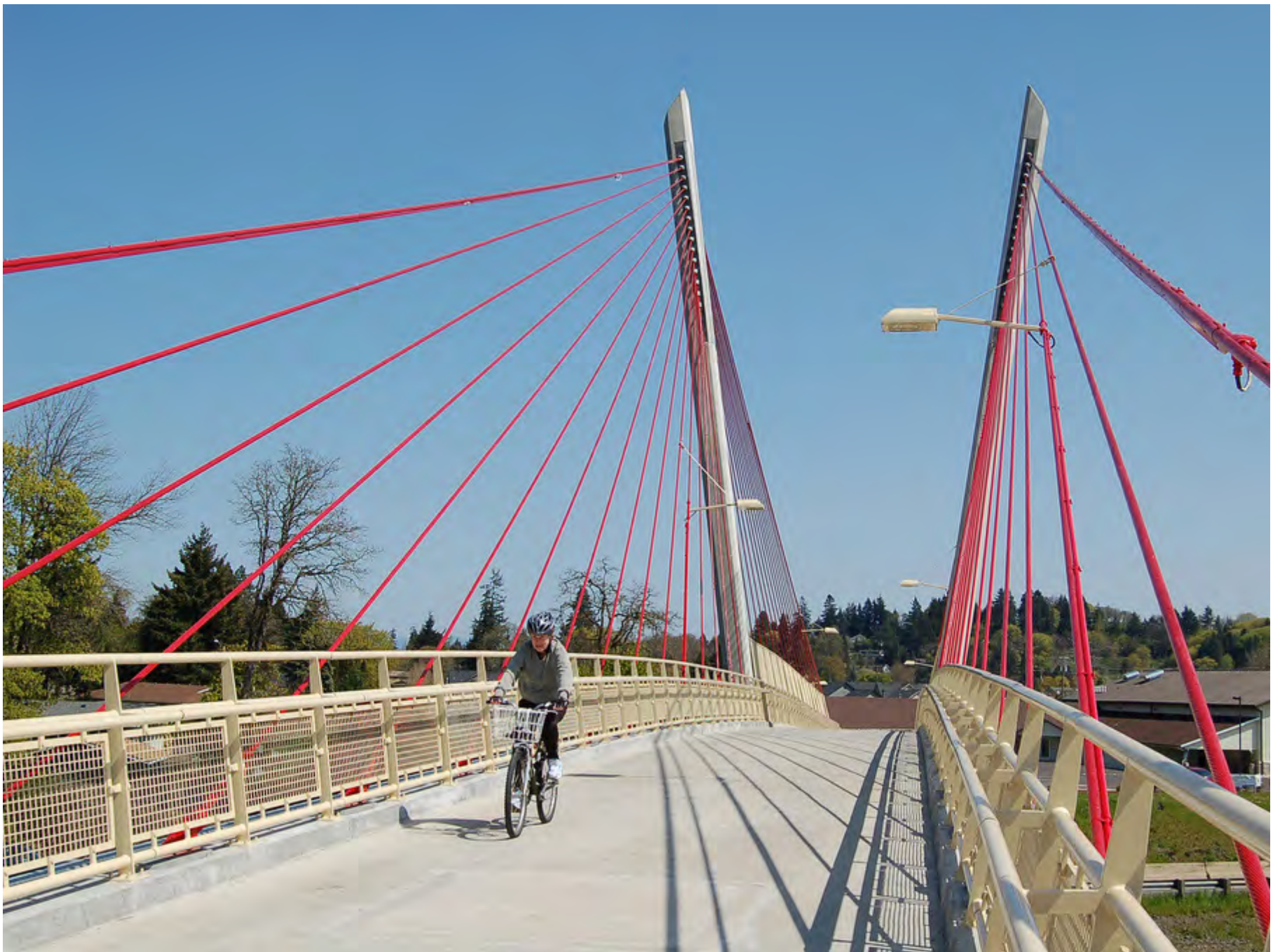
DELTA PONDS BRIDGE CABLE STAYED 14 FOOT CLEAR WIDTH EUGENE, OR
