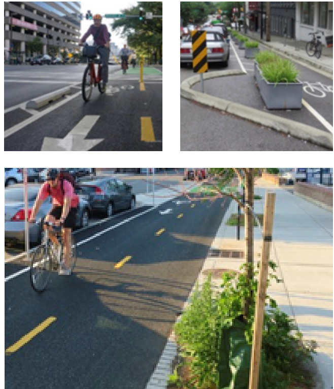
Figure 1.49: Protected bike lanes (Kirkland Design Guidelines).
