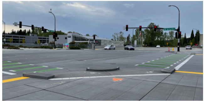
Figure 1.52: Protected intersection in Bellevue (City of Kirkland).
