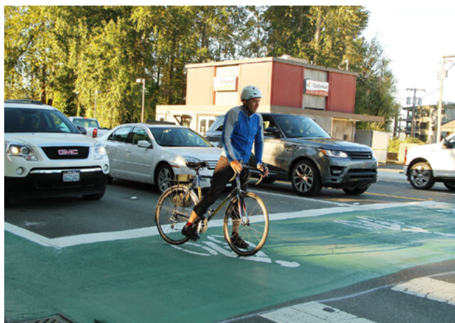
Figure 1.61: Bicycle queue box near Juanita Village (City of Kirkland).
