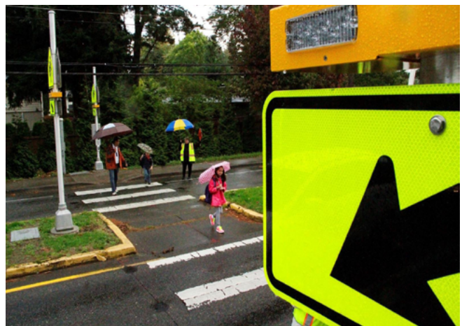
Figure 1.27: RRFB crossing with median refuge island at NE 116th St near Alexander Graham Bell Elementary School (City of Kirkland).
