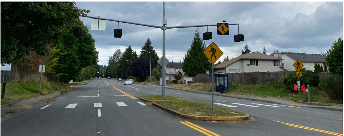
JN 16 Enhance Crossing: NE 124th St at 108th Ct NE
