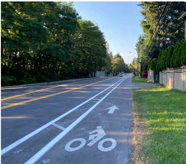
SRH 08 Sidewalk: 116th Ave NE from north of NE 75th Pl to south of NE 75th
