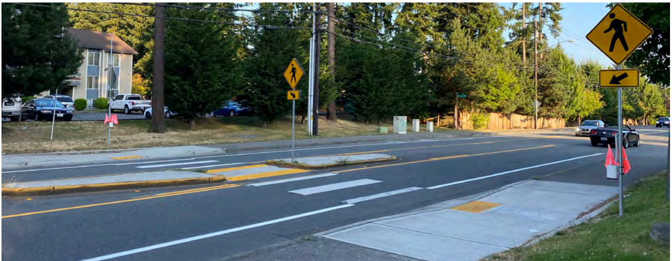
EH 09 Enhance crossing: 124th Avenue NE at NE 143rd Street
