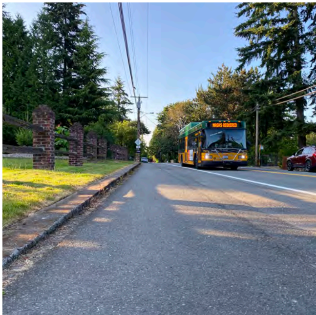
NRH 02 Sidewalk: 132nd Avenue NE from NE 110th Place to NE 97th Street
