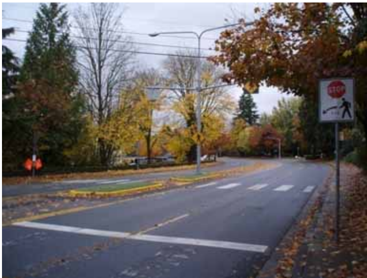
Figure 24 Crosswalk near the Casa Juanita senior housing facility. The crosswalk improvement program funded new islands, lighting and signing.
