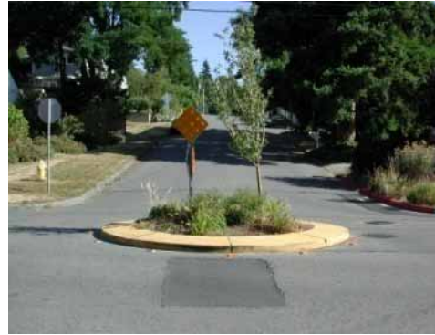
Figure 31 Traffic calming devices in neighborhoods slow traffic but sometimes require cyclists and drivers compete for the same space.
