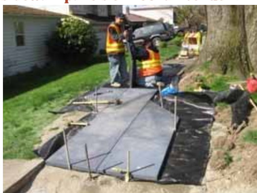
Figure 20 Installation of rubber sidewalk panels on 103rd Avenue NE
