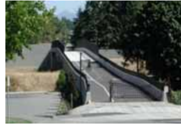
Figure 4 This bridge over I-405 at NE 100th Street helps tie neighborhoods together
