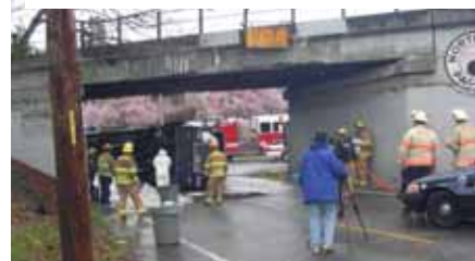
Figure 10 Railroad bridge at Kirkland Way. This low and narrow bridge is difficult for cyclists, walkers and tall vehicles.
