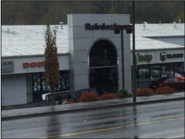
Figure 7-110. 12828 NE 124 th St., view northeast.
