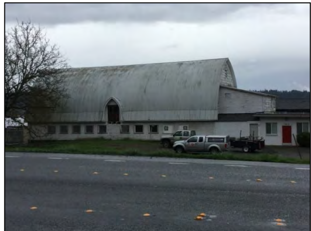
Figure 7-129. Barn at 12210 Willows Rd. NE, view east.
