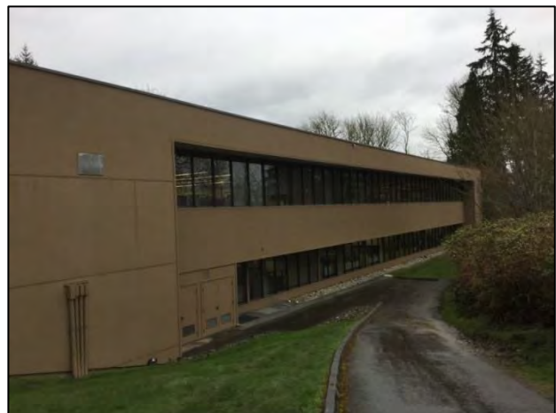
Figure 7-136. 11811 Willows Rd. NE, view southeast.
