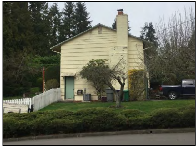
Figure 7-50. 12805 109 th Ave. NE, view north.
