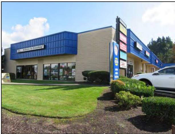
Figure 7-156. 13205 NE 124 th St., view south.
