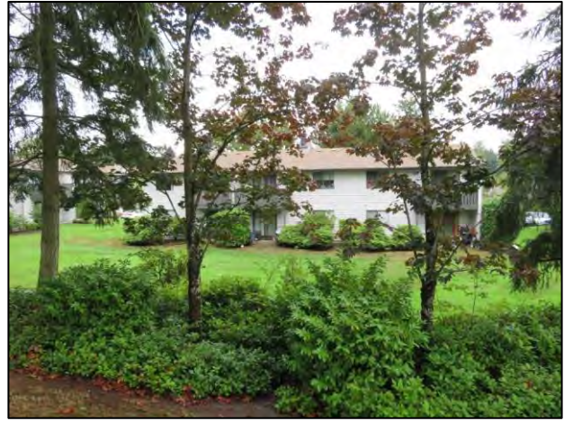
Figure 7-142. Emerson Apartment complex at 11010 NE 124 th Pl., view north.
