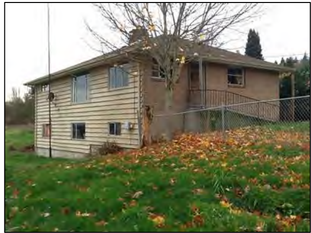
Figure 7-127. House at 12210 Willows Rd. NE, view southwest. Image courtesy of the King County Department of Assessments.
