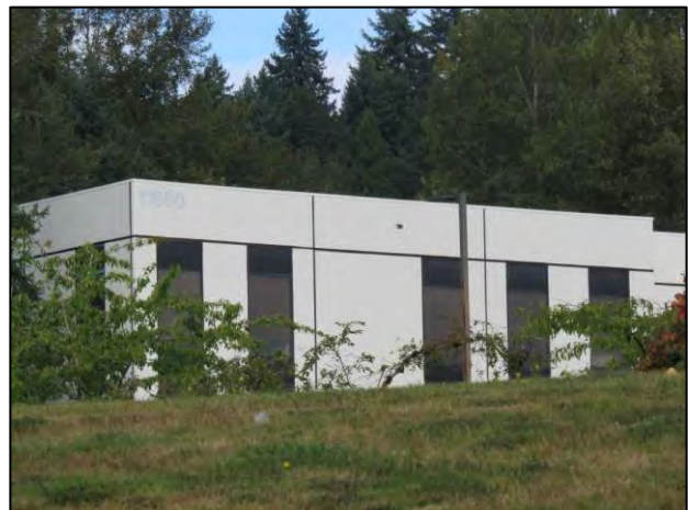
Figure 7-166. 11650 139 th Pl. NE, view northwest.
