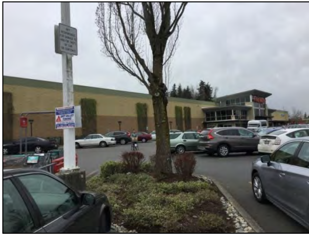
Figure 7-83. 12221 120 th Ave. NE, view northwest.
