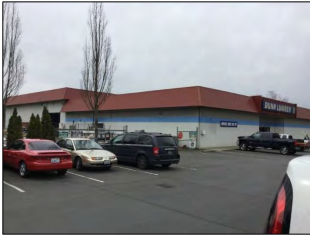
Figure 7-86. 11835 120 th Ave. NE, view northwest.
