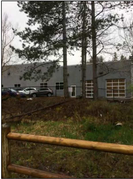
Figure 7-114. 12415 Slater Ave. NE, view south.
