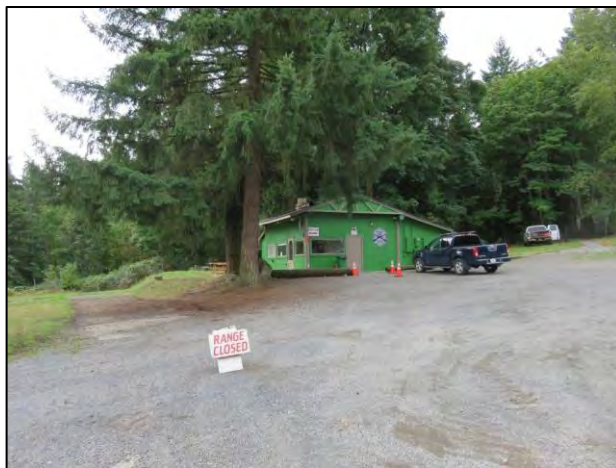
Figure 7-174. 13633 NE 97 th St., shooting range and clubhouse or skeet building, view south.
