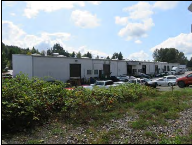
Figure 7-178. 12706 NE 124 th St., view southwest.
