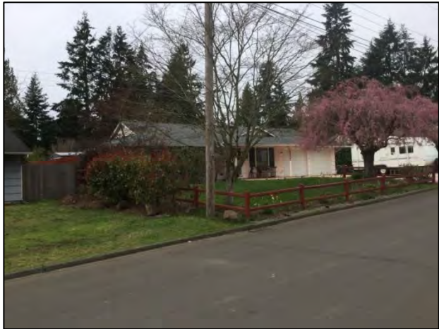
Figure 7-67. 12829 110 th Ave. NE, view northwest.
