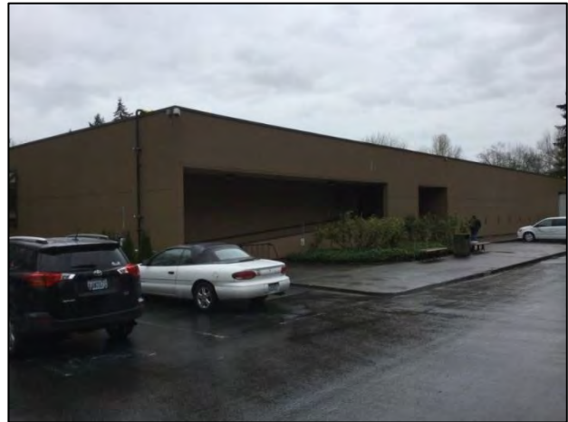
Figure 7-134. 11811 Willows Rd. NE, view southwest.
