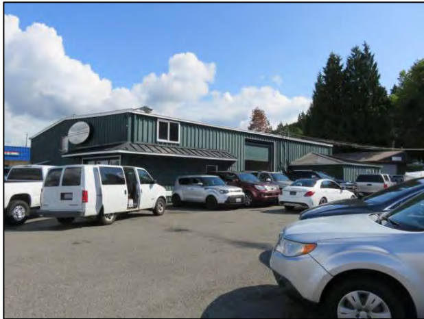
Figure 7-155. 13131 NE 124 th St., view southeast.
