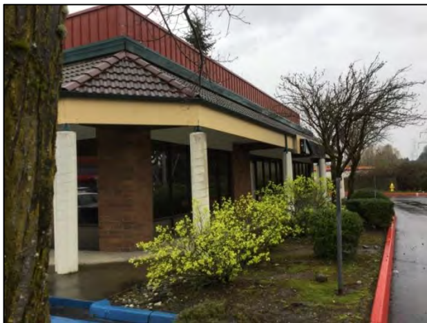
Figure 7-100. 11961 124 th Ave. NE, view northwest.
