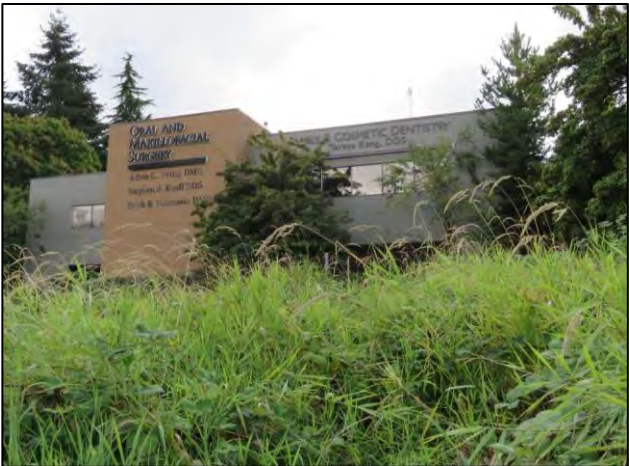
Figure 7-147. 12330 120 th Ave. NE, view south.
