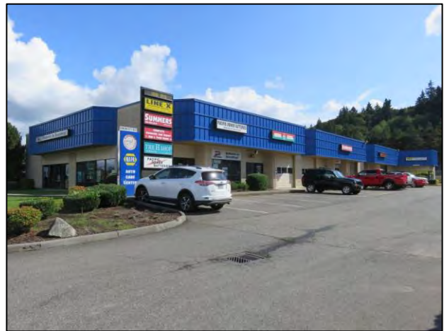
Figure 7-157. 13205 NE 124 th St., view southeast.
