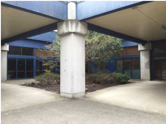
10601 NE 132ND ST, courtyard
