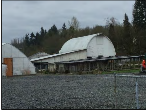
Figure 7-130. Barn at 12210 Willows Rd. NE, view southwest.
