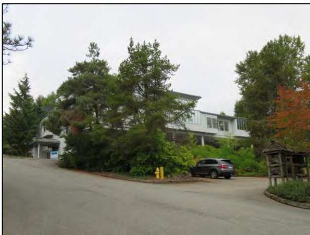
Figure 7-160. 12515 Willows Rd. NE, view west.
