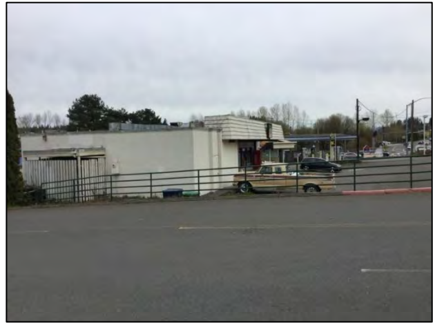
Figure 7-75. 11438 NE 124 th St., view northeast.
