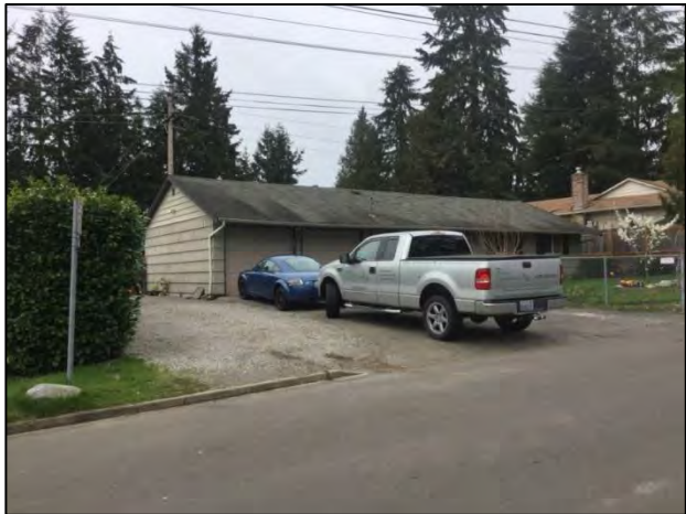
Figure 7-65. 12835 110 th Ave. NE, view northwest.
