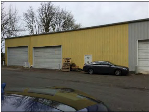
Figure 7-91. 11731 120 th Ave. NE, view northwest.
