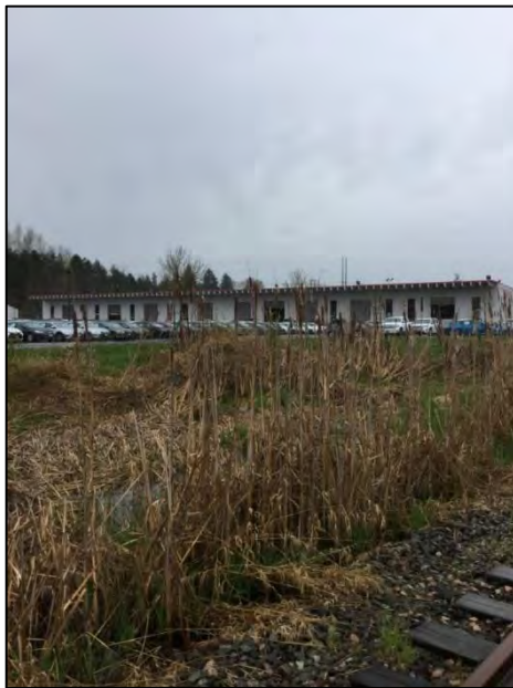
Figure 7-119. 13225 NE 126 th Pl., view northeast.
