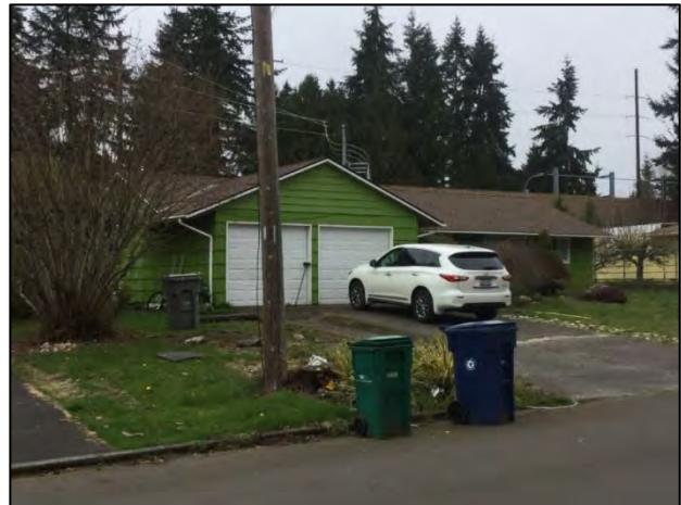
Figure 7-55. 13025 110 th Ave. NE, view northwest.
