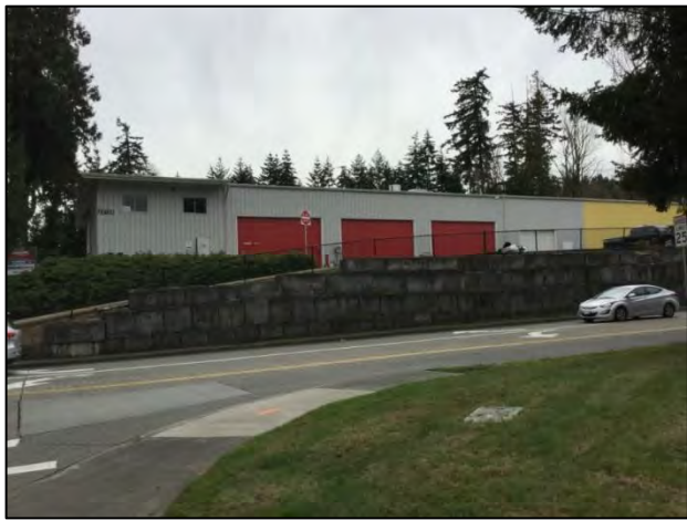
Figure 7-89. 11731 120 th Ave. NE, view south.
