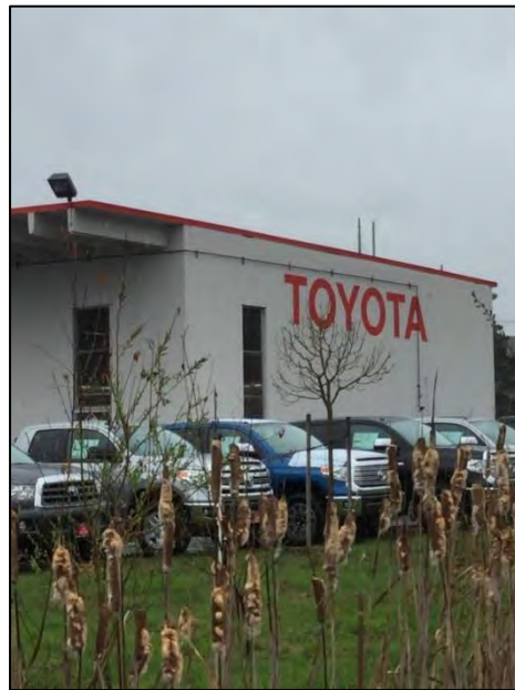
Figure 7-120. 13225 NE 126 th Pl., view northeast.
