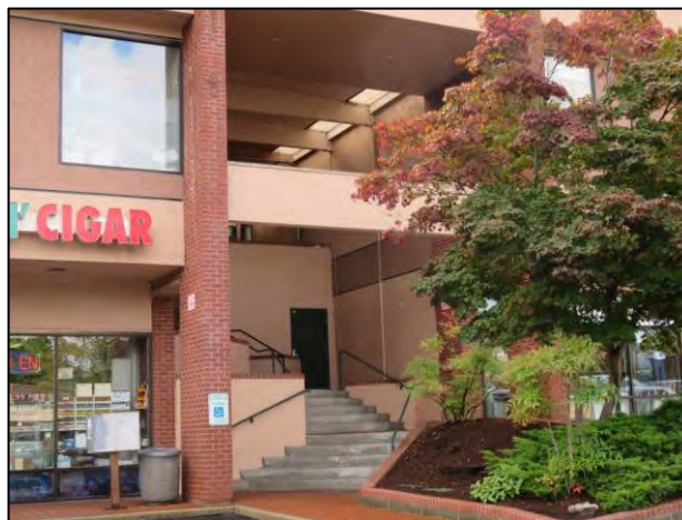
Figure 7-145. The breezeway, Totem Lake West at 11410 NE 124 th St., view south.
