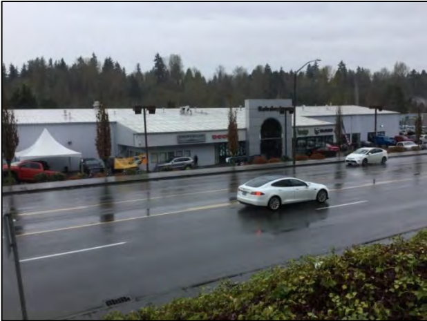
Figure 7-109. 12828 NE 124 th St., view northeast.
