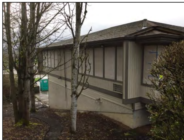
Figure 7-125. 12525 Willows Rd. NE, view southeast.
