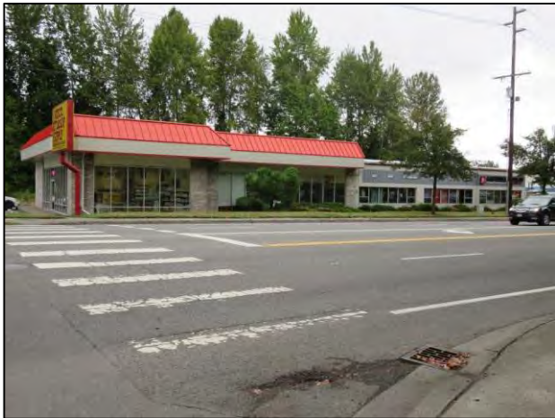
Figure 7-152. 13400 NE 124 th St., view northeast.
