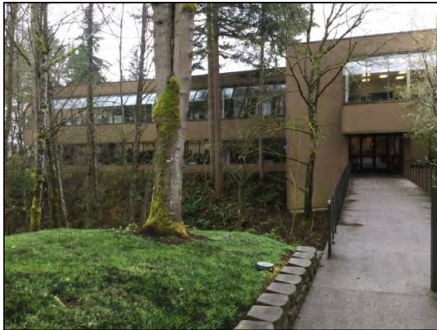
Figure 7-133. 11811 Willows Rd. NE, view west.
