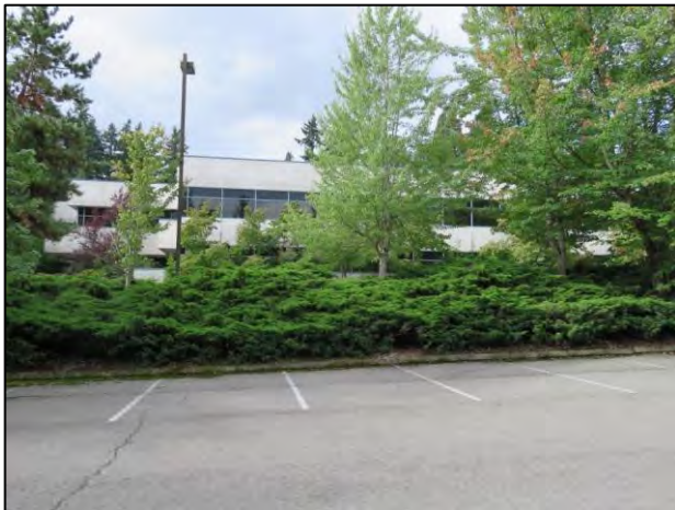
Figure 7-167. 10301 Willows Rd. NE, view west.
