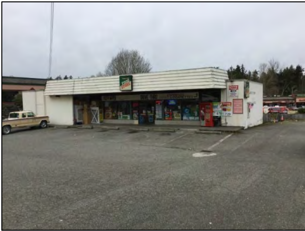
Figure 7-74. 11438 NE 124 th St., view northwest.
