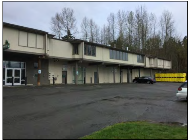
Figure 7-124. 12525 Willows Rd. NE, view northwest.
