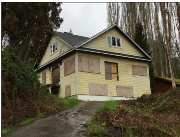
Figure 7-131. 12195 Willows Rd. NE, house, view northwest.
