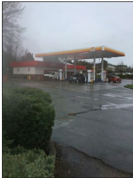
Figure 7-92. 12221 124 th St. NE, view southwest.
