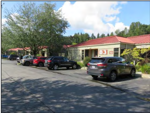
Figure 7-148. 12509 130 th Ln. NE, view northwest.
