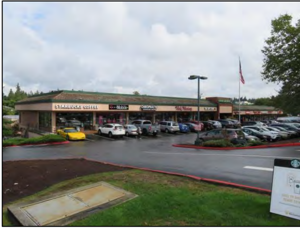
Figure 7-143. Totem Lake West at 11410 NE 124 th St., view northeast.
