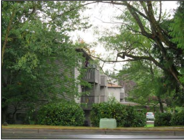
Figure 7-141. Emerson Apartment complex at 11010 NE 124 th Pl., view north.
