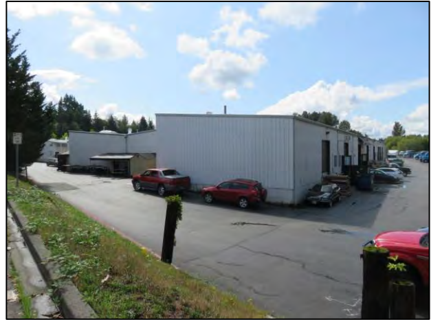
Figure 7-179. 12706 NE 124 th St., view west.
