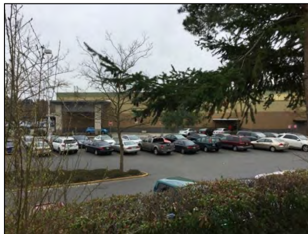
Figure 7-85. 12221 120 th Ave. NE, view south.
