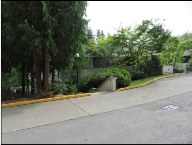
Figure 7-169. 10201 Willows Rd. NE, view southeast.
