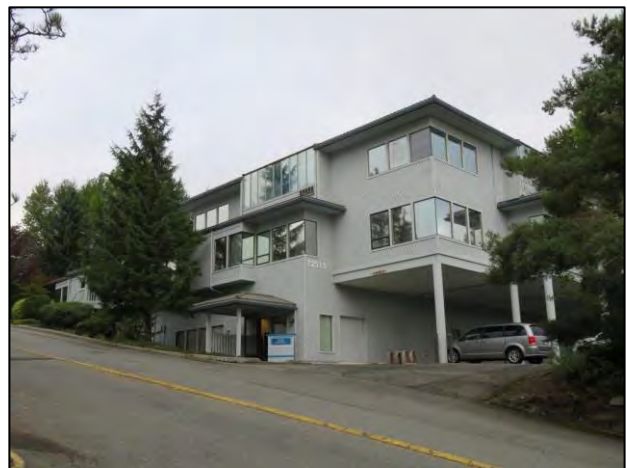
Figure 7-161. 12515 Willows Rd. NE, view northwest.
