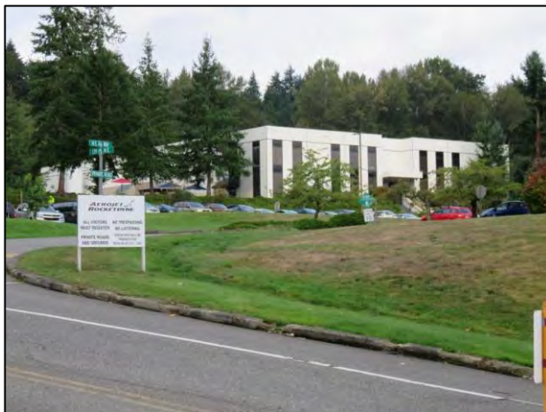
Figure 7-165. 11650 139 th Pl. NE, view northwest.
