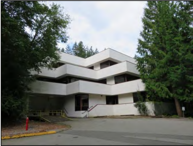
Figure 7-170. 10201 Willows Rd. NE, view north.
