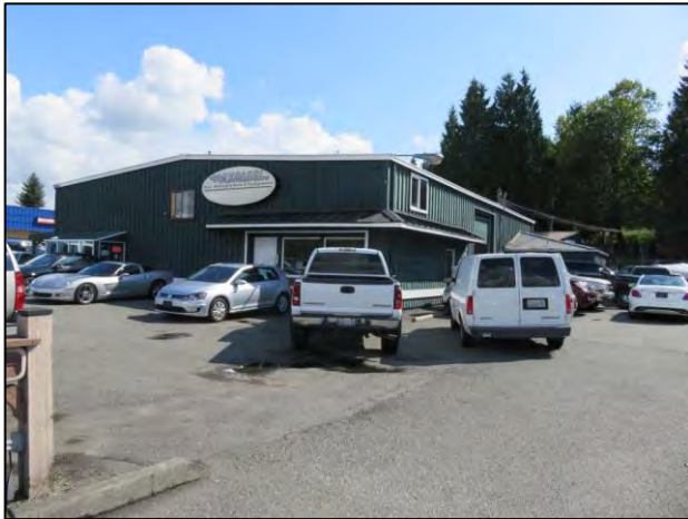
Figure 7-154. 13131 NE 124 th St., view southeast.
