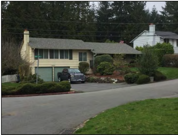
Figure 7-49. 12805 109 th Ave. NE, view northwest.
