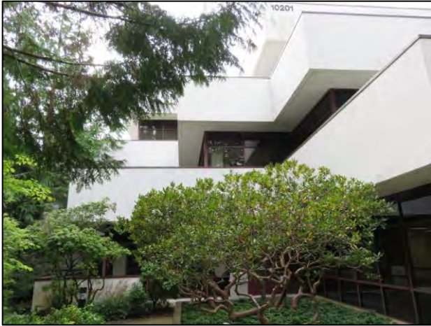
Figure 7-171. 10201 Willows Rd. NE, close-up of southern balconies, view west.
