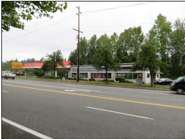
Figure 7-153. 13400 NE 124 th St., view northwest.
