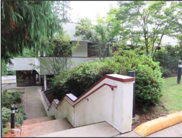
Figure 7-172. 10201 Willows Rd. NE, view of stair to secondary entry, view east.
