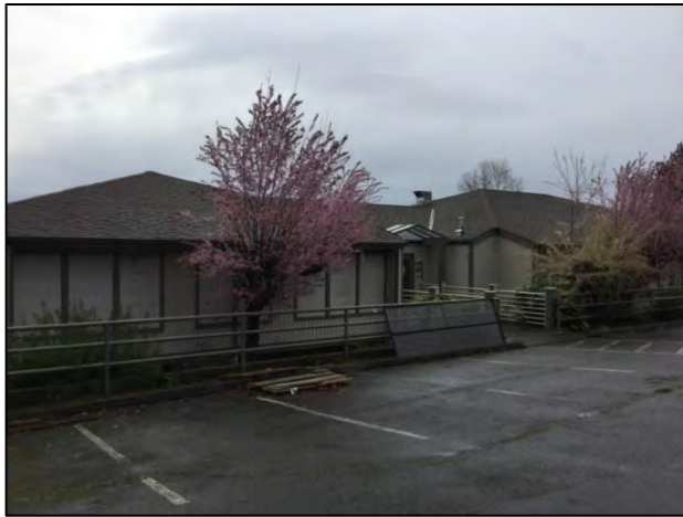
Figure 7-123. 12525 Willows Rd. NE, view southeast.
