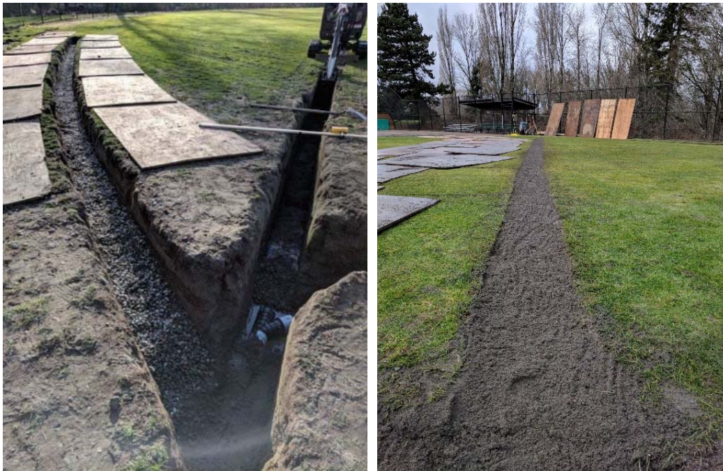
DRAINAGE IMPROVEMENTS TO CRESTWOOD FIELD #4
